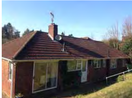
Plate 1: 153 Hemdean Road (eastern aspect) – building in good condition with very limited potential to support roosting bats.
