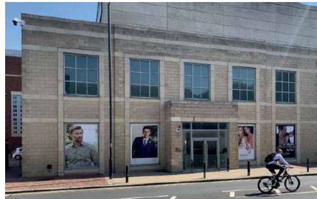
↑ The staff entrance has been constructed in a Georgian style
