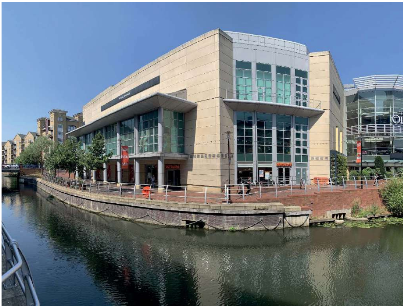
⬆ The corner 'splay' element consists of full height glazing
