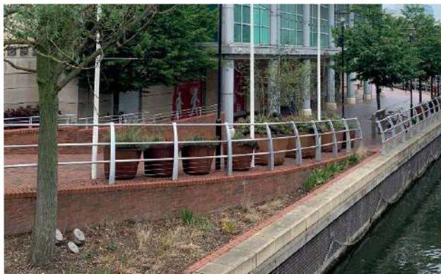
↑ Parts of the soft landscape have suffered during the hot summer
