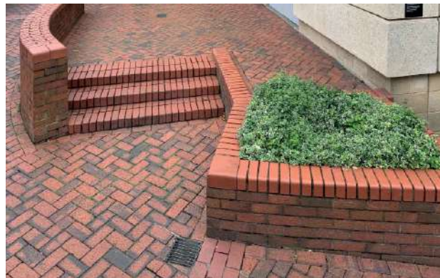
↑ Hard landscape is constructed from red/grey block paving
