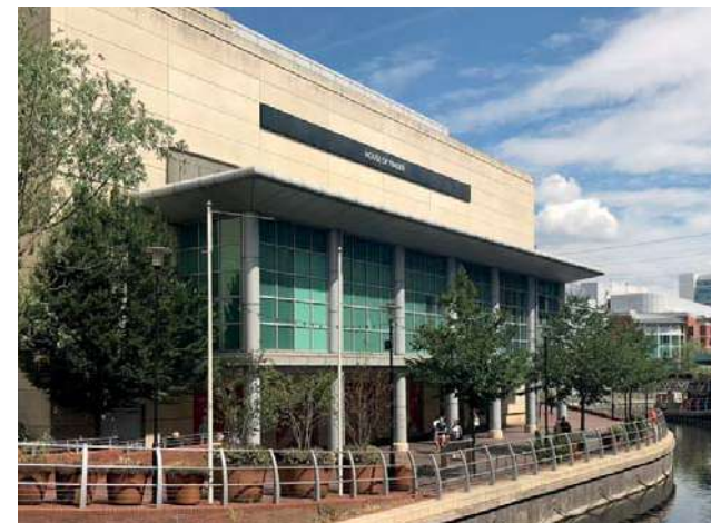
⬆ The 'pop out' element forms a colonnade along the Riverside
