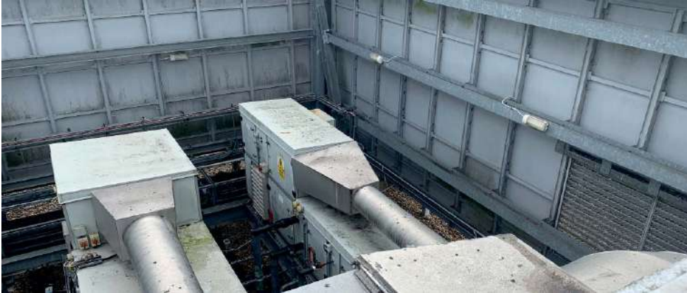
Plant areas are shielded by 4m high plant screens which are set back from the building line
