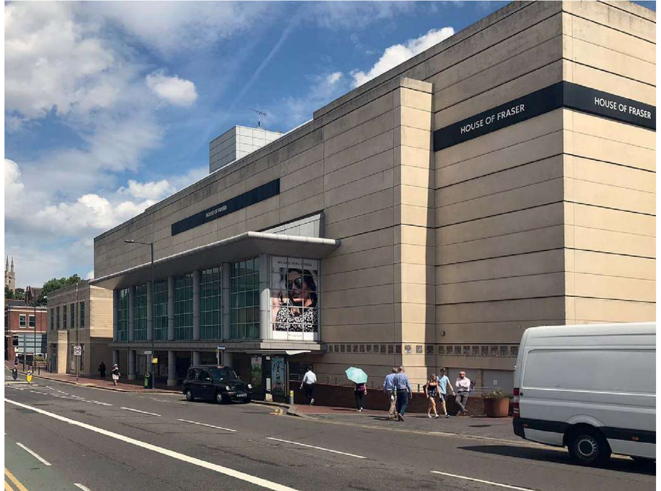
📍 The Bridge Street façade also includes a 'pop out' feature
