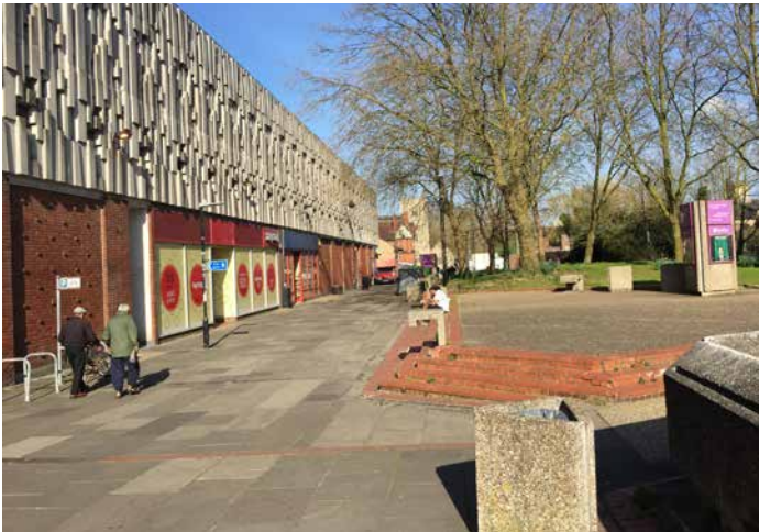
Broad Street Mall Car Park Concrete Facade
