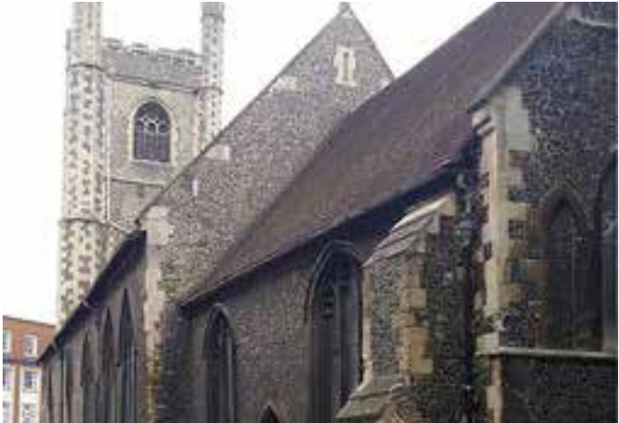
St Laurence Church Flint with Ashlar Quoining
