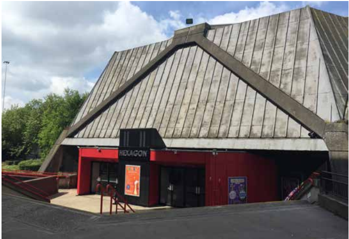
Hexagon Theatre - Zinc Panelling
