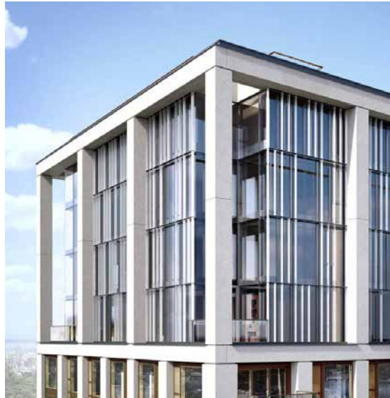
Casson Square - Squire & Partners (Under Construction)
