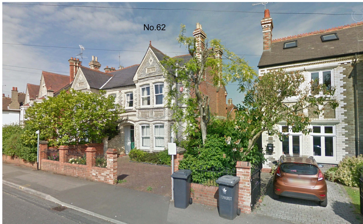
No.62 Front Elevation [Elmhurst Road]
