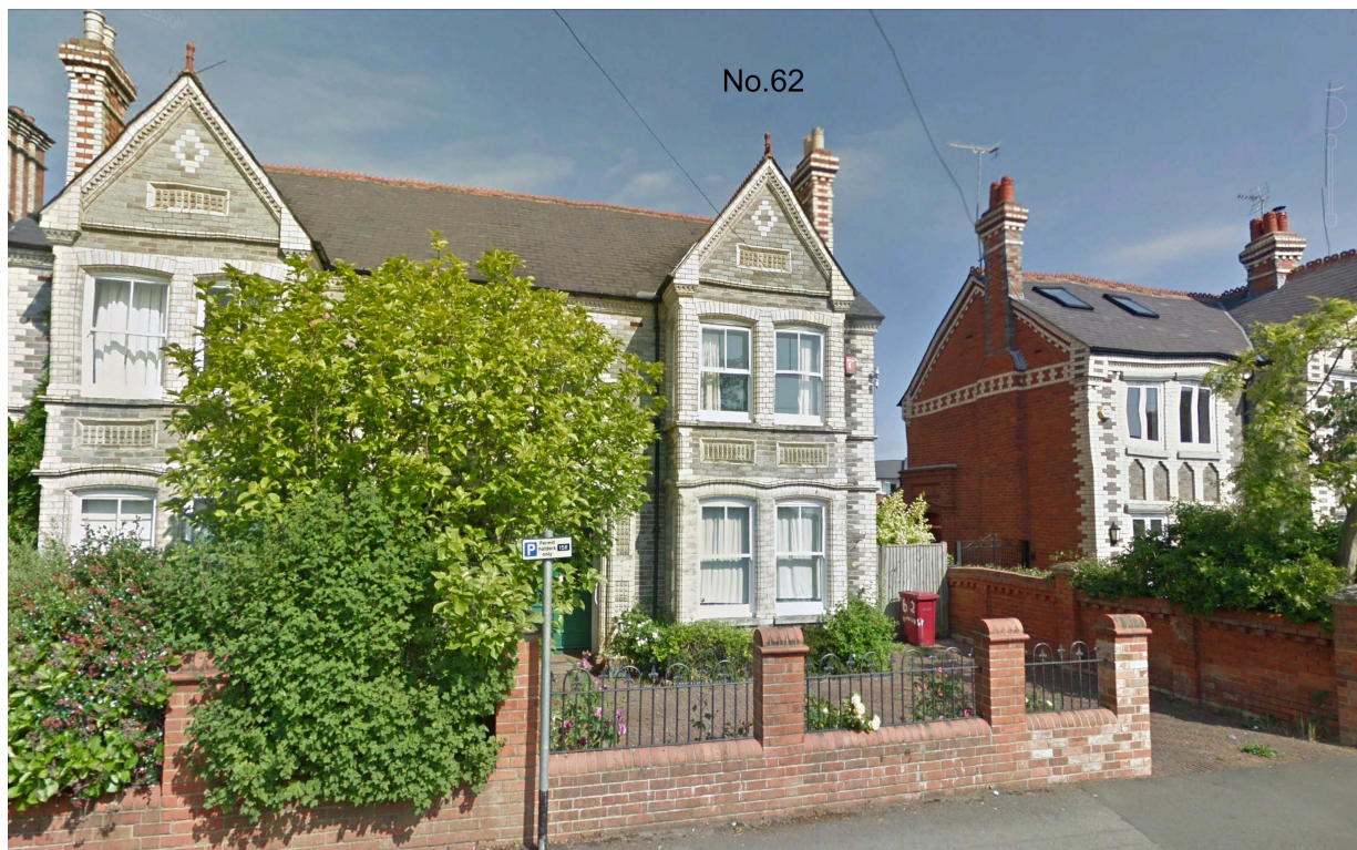
No.62 Front Elevation [Elmhurst Road]
