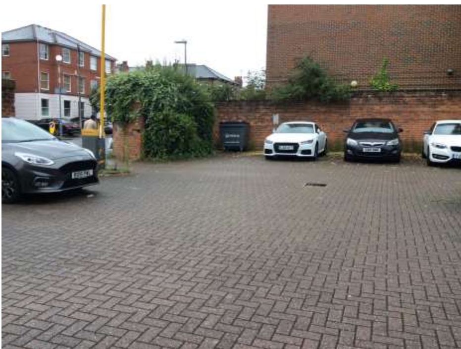
Photo 19. Brick wall on Southern boundary
