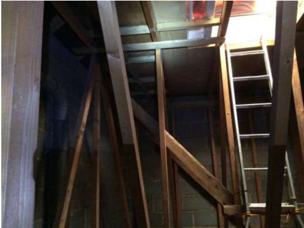
Photo 5. B58 loft space
