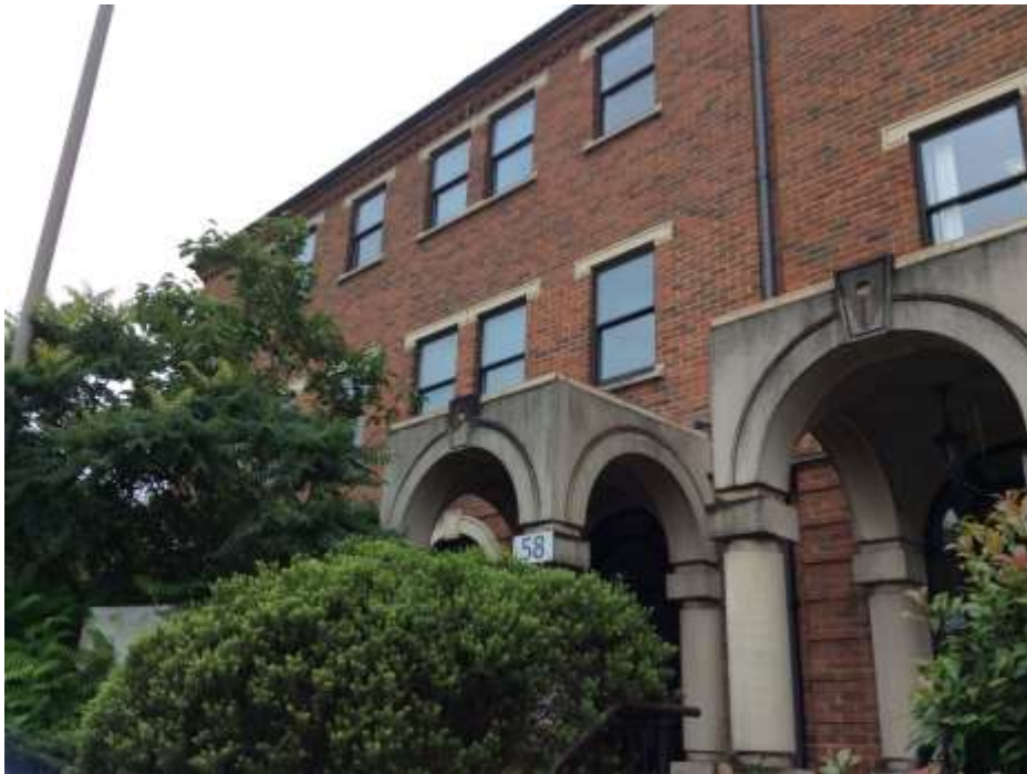
Photo 1. B58, front view, Northern face
