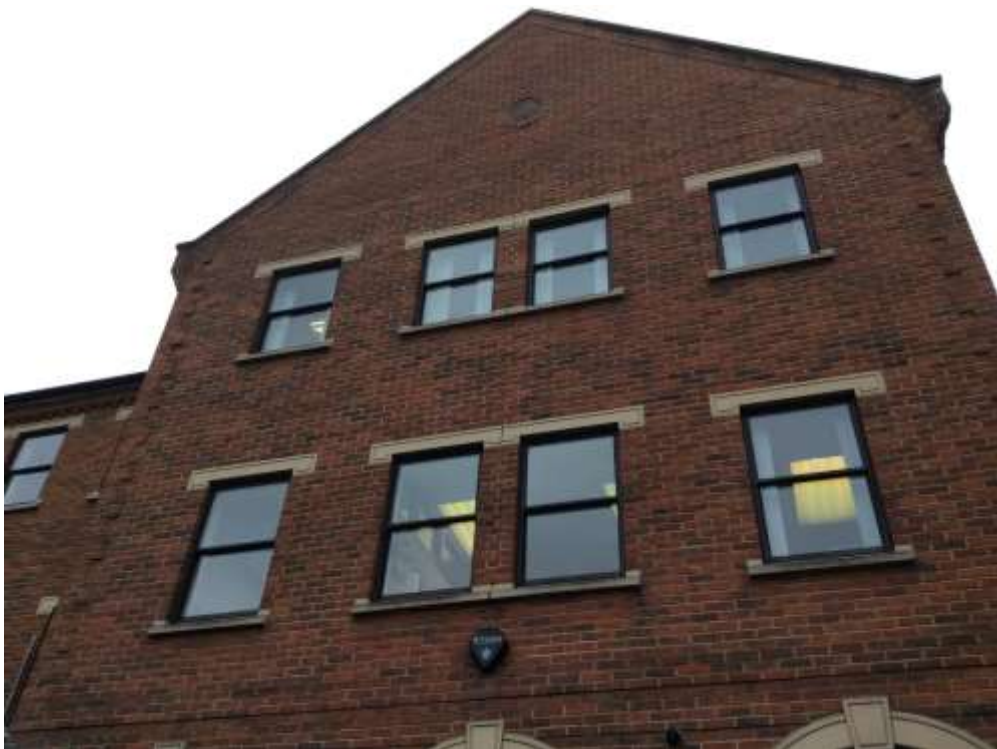
Photo 12. B54 front view, Northern face
