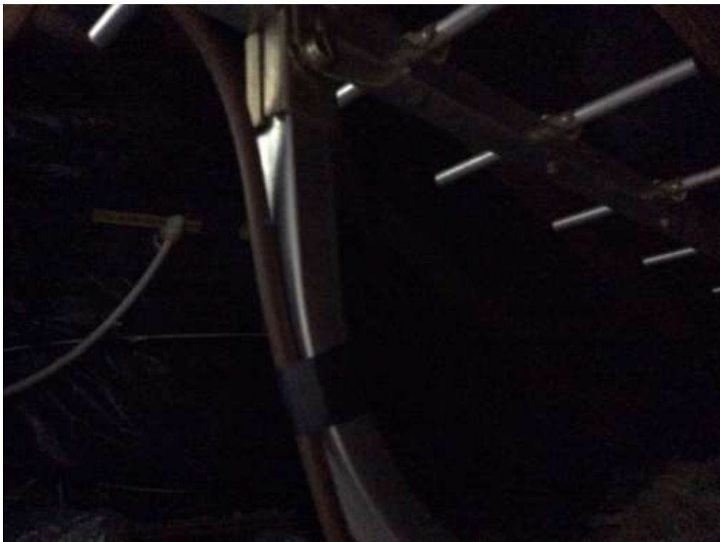
Photo 14. B54 loft space
