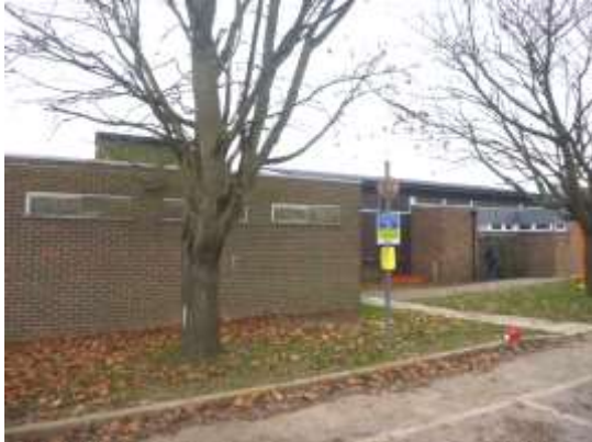
1. Front of the pavilion viewed from the north
