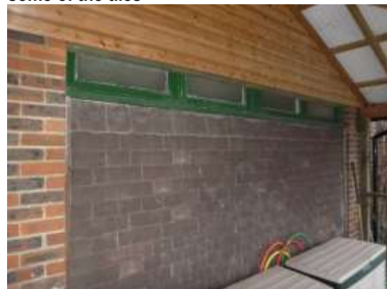
12. Hanging tiles under the canopy to the eastern side of the pavilion
