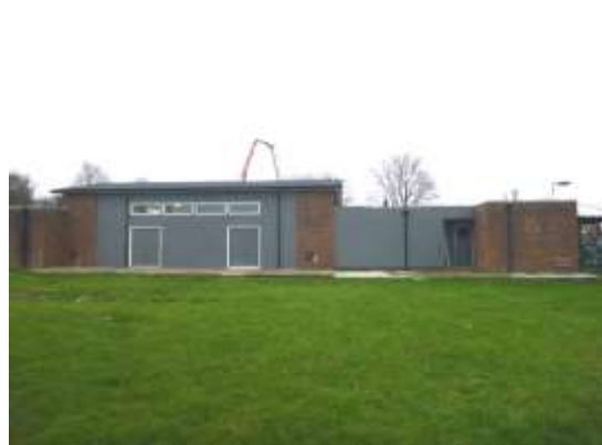
2. Rear of the pavilion viewed from the south
