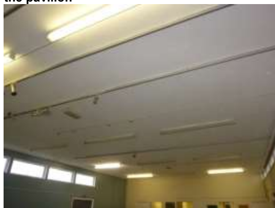
18. Internal view of the main central pitched roofed section of the pavilion with no access to a roof space
