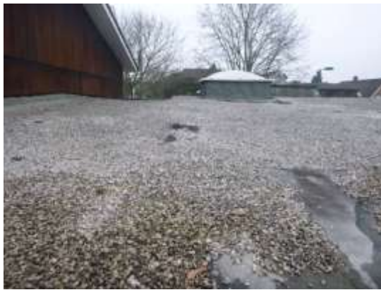
7. Flat roof at eastern end of the building covered tightly with bitumen felt and gravel
