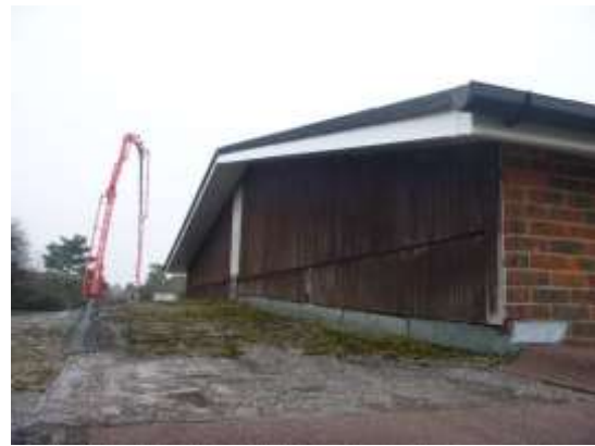
8. Flat roof at western end of the building covered tightly with bitumen felt and gravel
