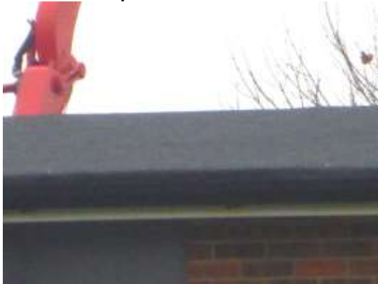
3. The central pitched roof tightly covered with bitumen felt
