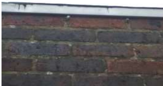
9. Metal trim tight around the flat roof
