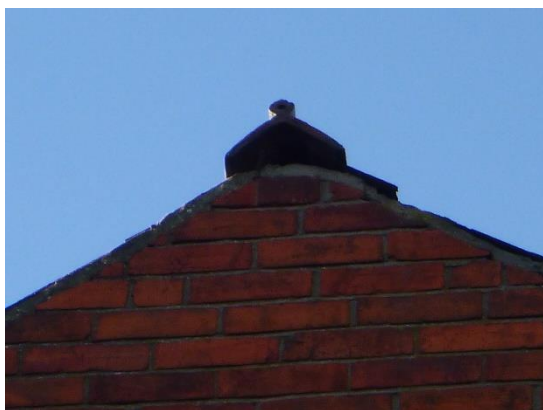
7. Ridge open at the gable end (eastern elevation).
