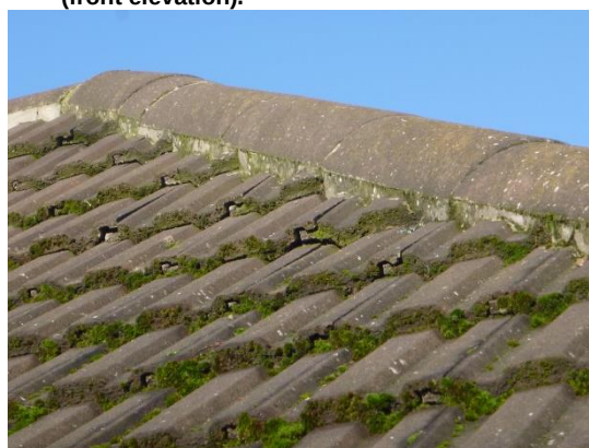
18. Hip tiles with mortar intact (front elevation).
