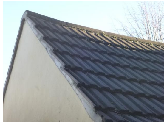
20. Verge mortar at rear gable end intact (rear elevation).
