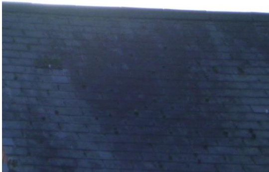
3. Overlapping slate tiles mostly flat and tightly fitted (rear elevation).
