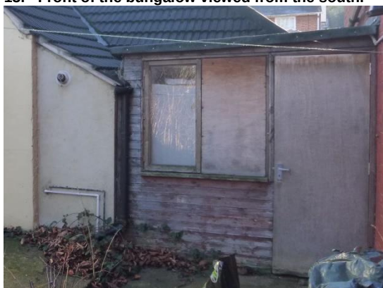
15. Timber extension joining to the end terraced house (rear elevation).
