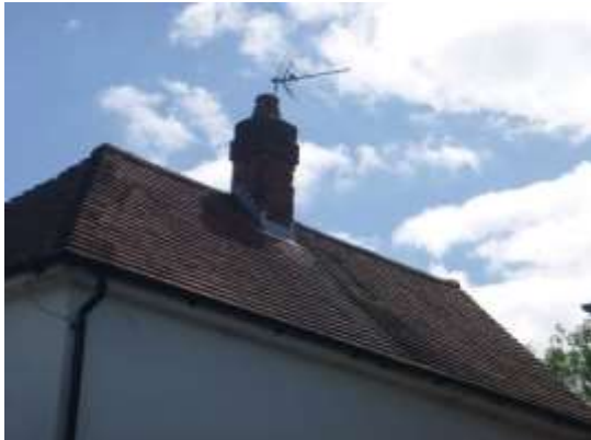
3. Tight roof tiles and lead flashing around the chimney (southwest elevation).
