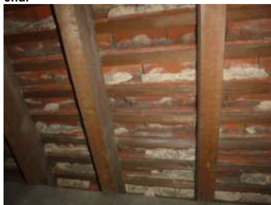
10. The unlined roof.
