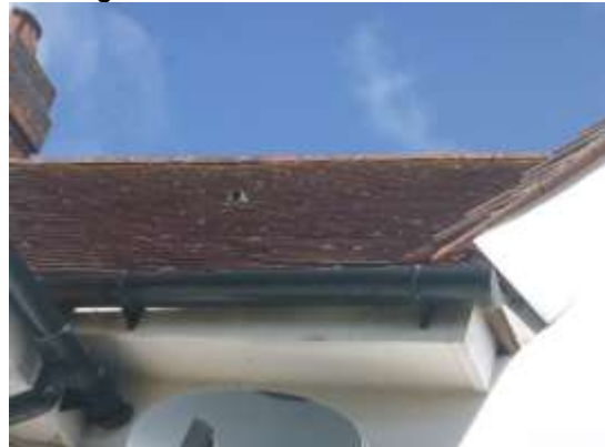
6. Intact mortar under the ridge on the front elevation.
