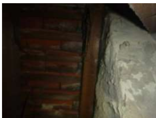
12. Unlined tiles around the chimney.
