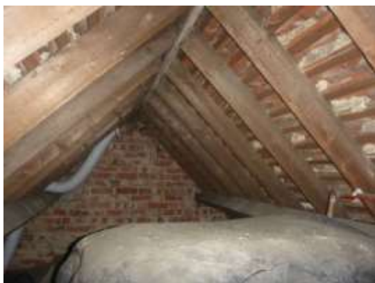
9. Roof space looking towards the rear gable end.
