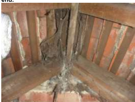
11. The cobwebbed ridge beam.
