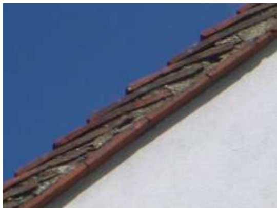
7. Intact verge mortar at the gable ends.
