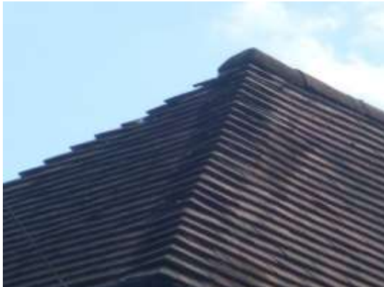
5. Intact mortar under the hip tiles.
