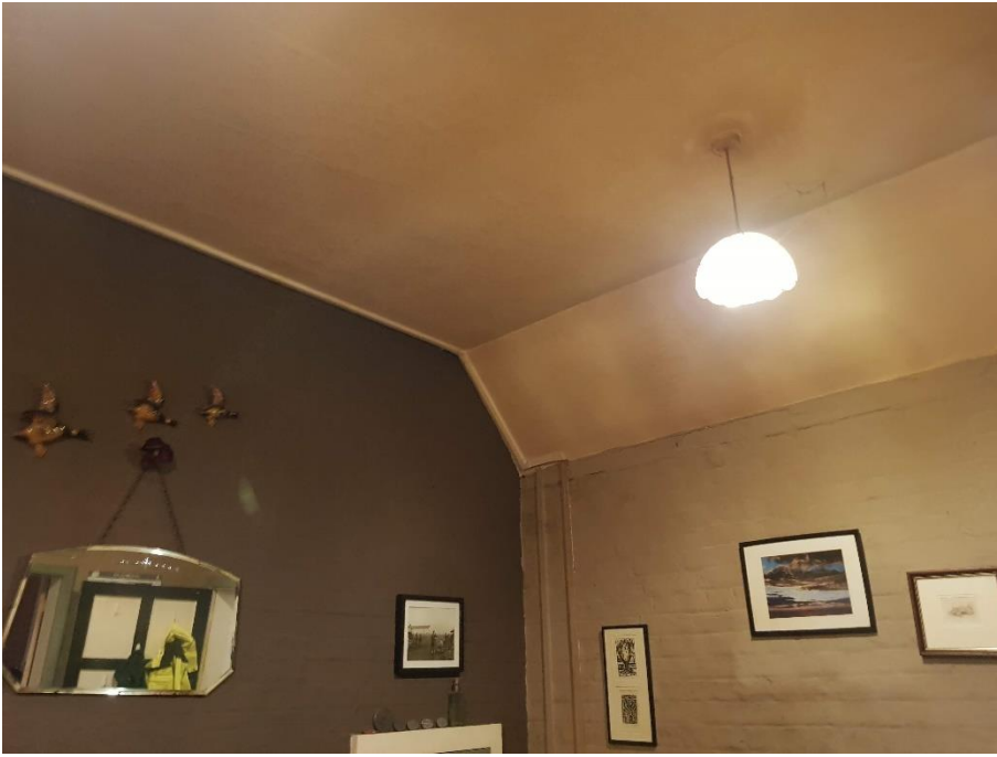
Figure 5 - Skeilings and external walls to be boarded over with insulation backed plasterboard
