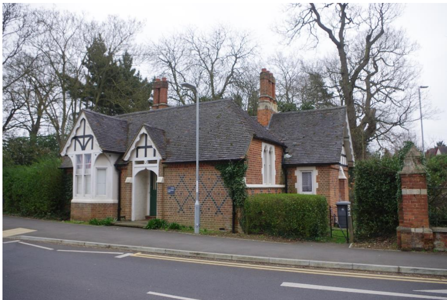
Figure 2 - General view of front elevation
