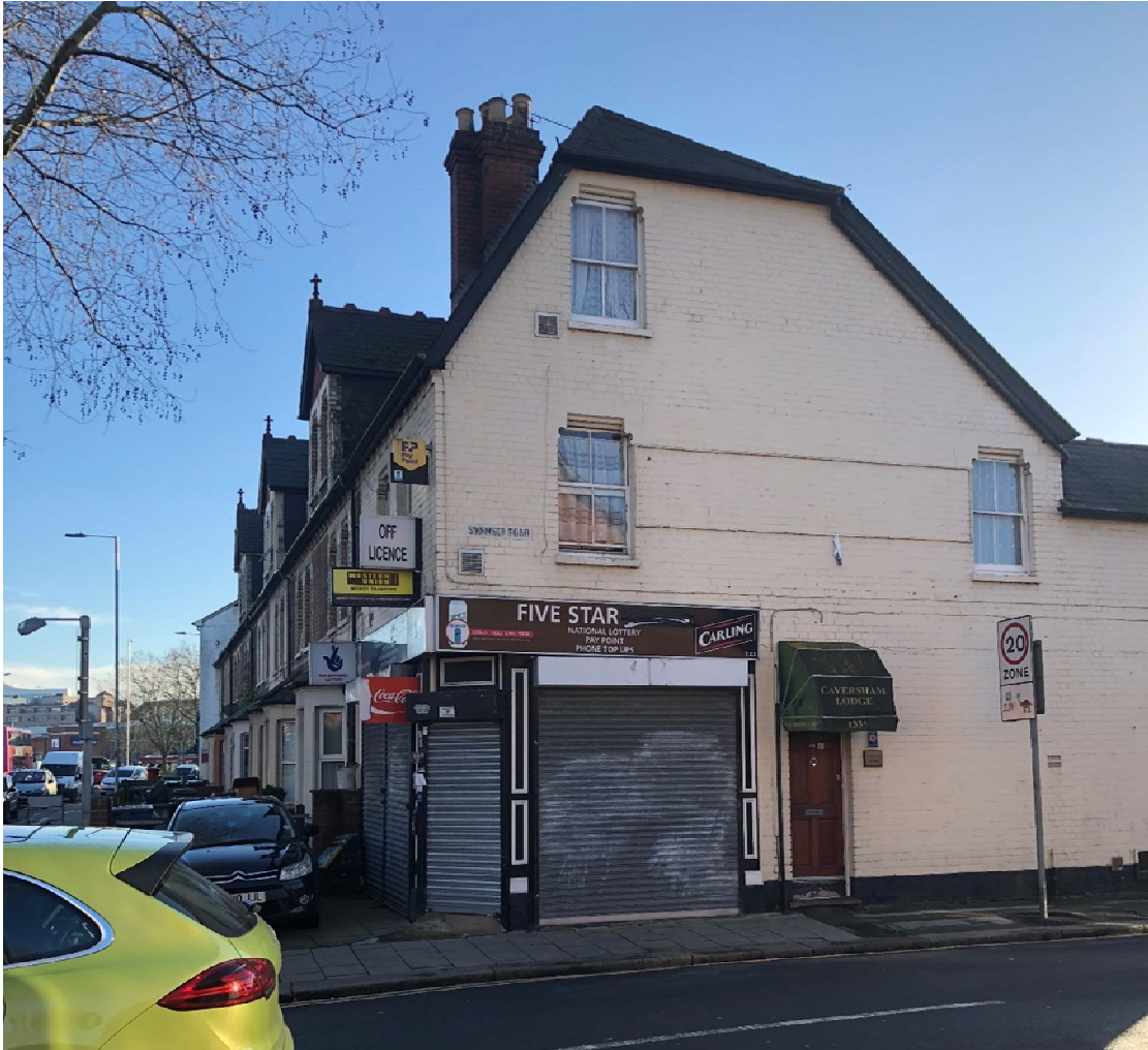
Fig.2 photo of the retail premises at No. 133 Caversham Road
