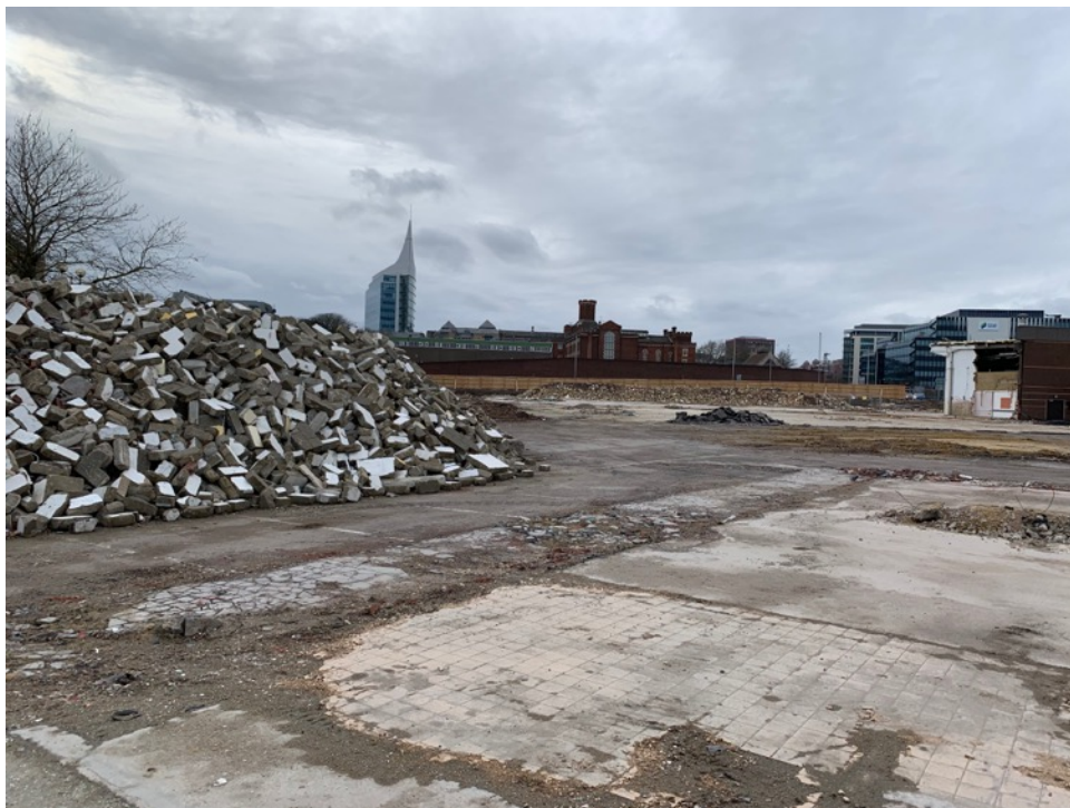
Photograph 4 Facing south-west showing stockpile of demolition material.
