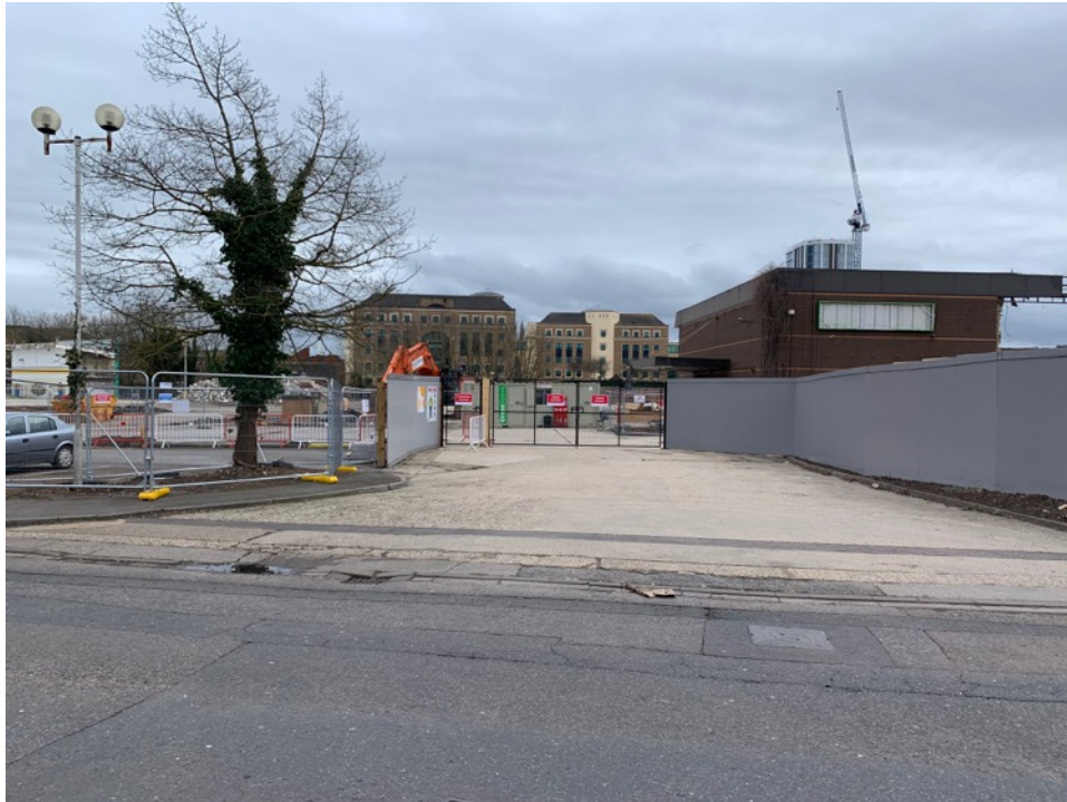
Photograph 1 Site entrance from Kenavon Drive.
