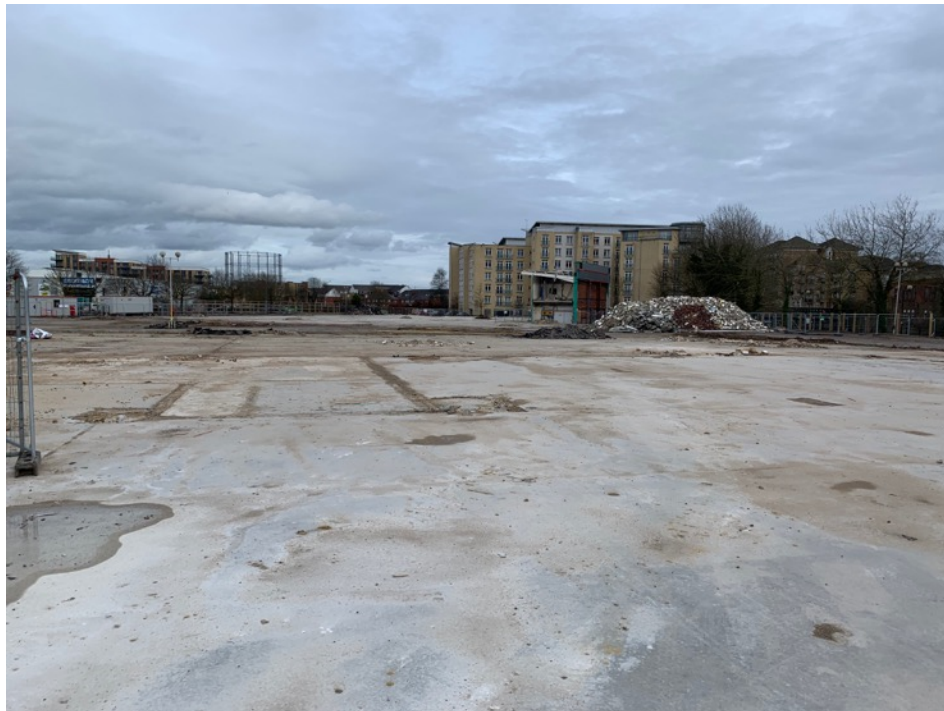
Photograph 5 Facing north-east showing extent of site at slab level.
