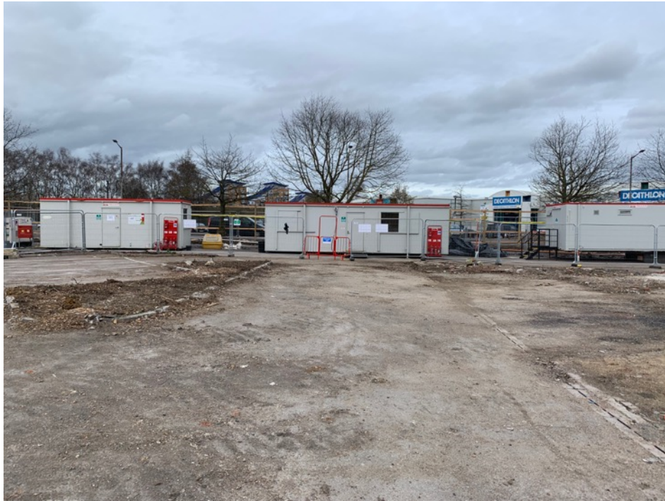
Photograph 3 Site compound area.
