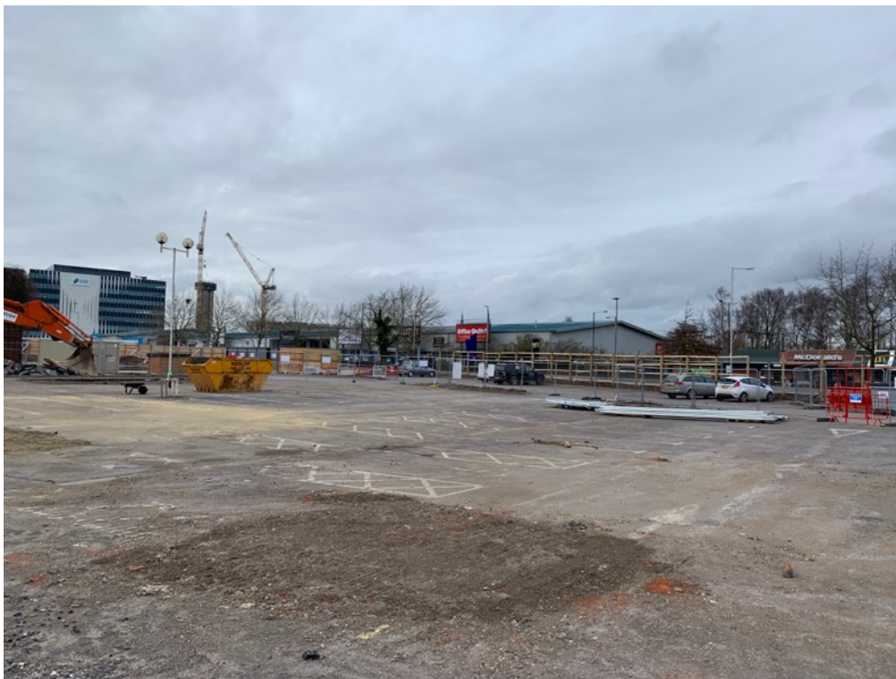
Photograph 2 Facing north-west showing northern extent of site, site compound and site parking area.
