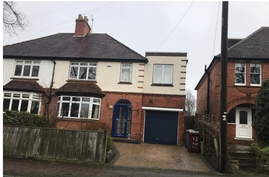
No.93 Northcourt Avenue
