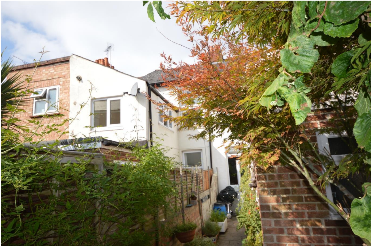
Pic. 2 Existing rear elevation
