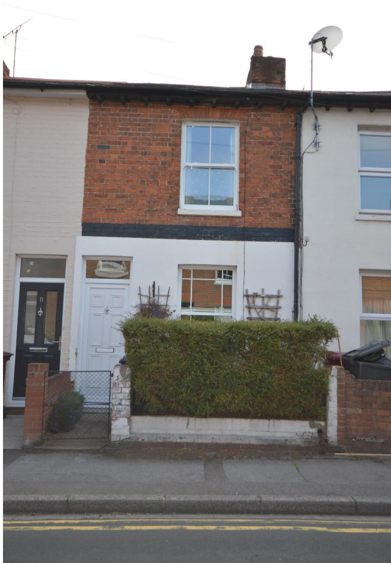
Pic.1 Front elevation of 13 Victoria Street, Reading
