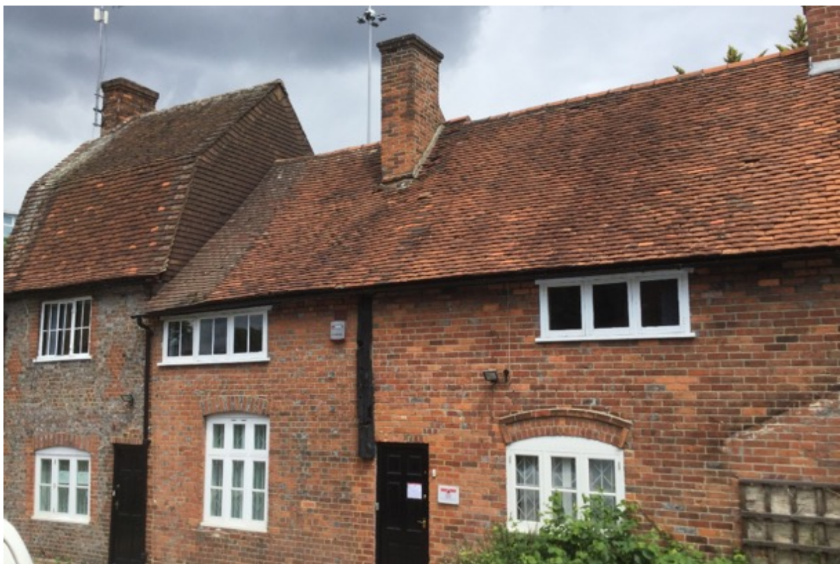
Photograph 2. The west facing elevation of the building at 26-28 Southampton Street.
