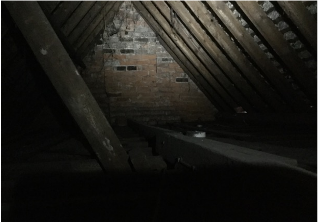
Photograph 3. The internal aspects of the confined, timber framed roof void at 26-28 Southampton Street.
