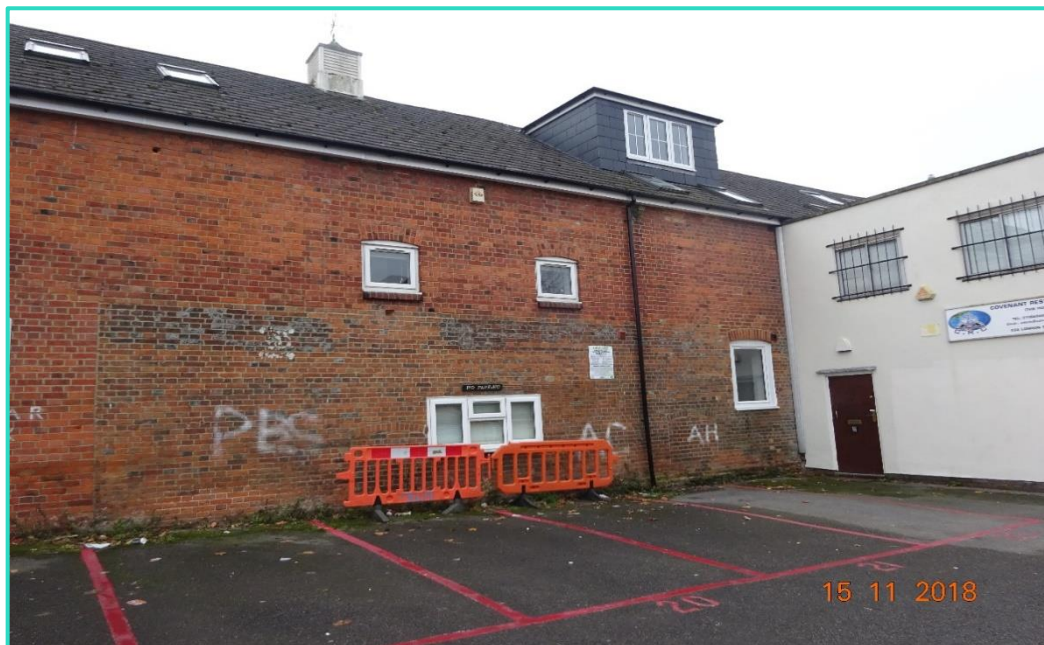
Extract 01: Site Photograph London Court W1/150, W1/160, W1/161 and W2/161
