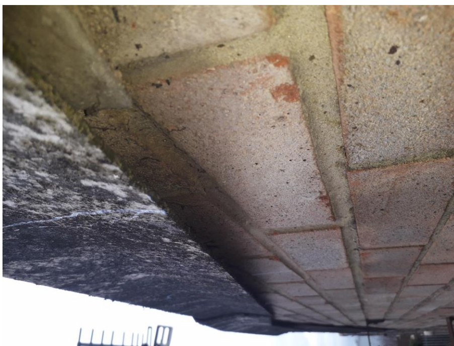
Figure 4.9 Gaps under roofing material
