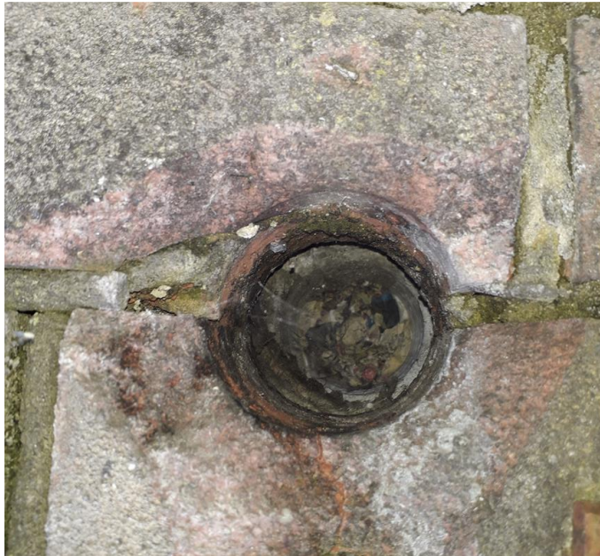
Figure 4.7 Hole in brickwork – old drain pipe
