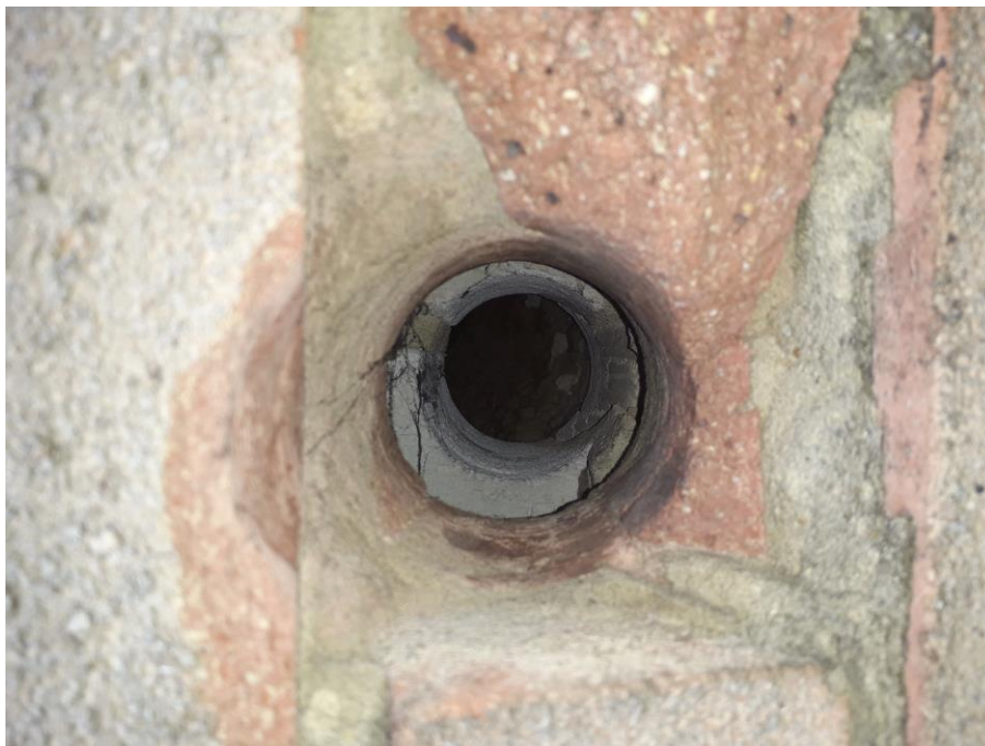
Figure 4.7 Hole in brickwork – old drain pipe
