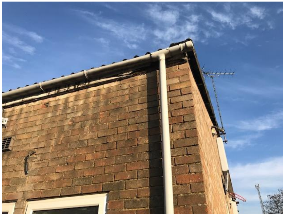
Figure 4.4 Rotten wooden fascia board on Building 4
