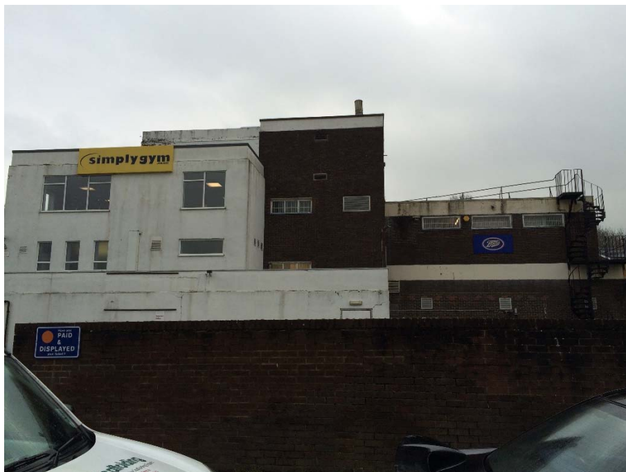
Photograph 4: South Elevation looking at Boots Retail and Health Club.
