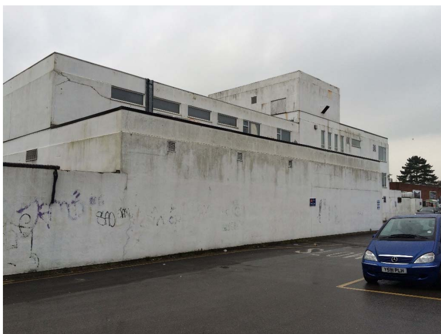
Photograph 5: West Elevation from the rear car park.
