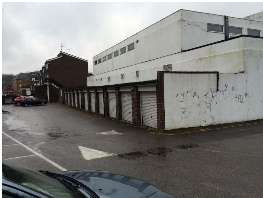
Photograph 6: Existing garages along north elevation.
