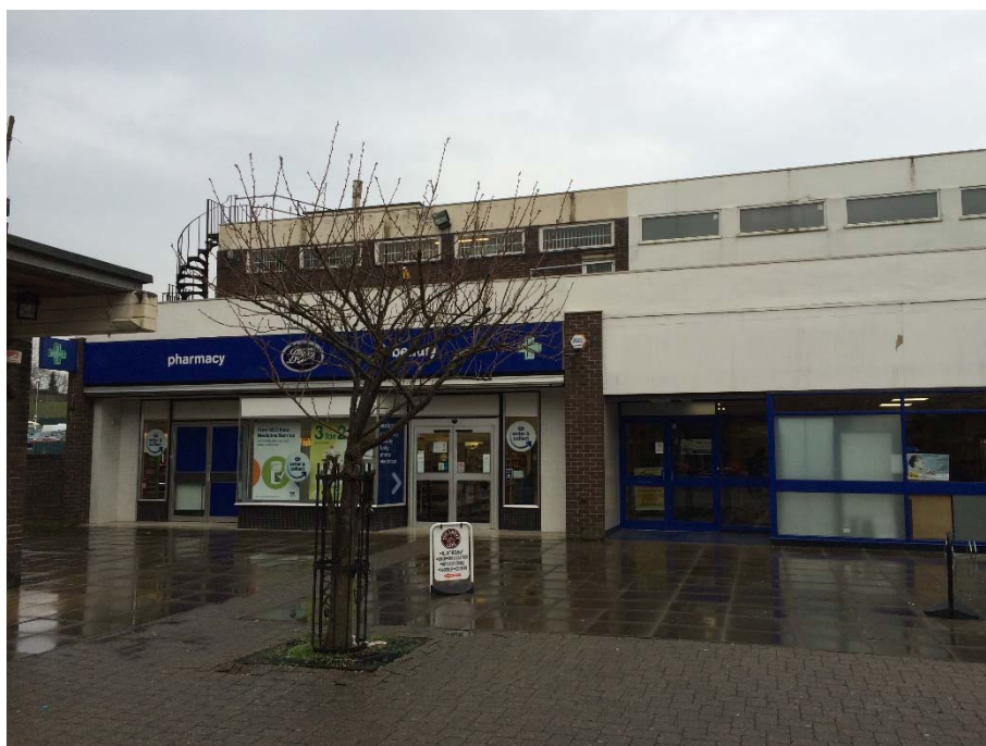
Photograph 1: Part East Elevation looking towards Boots Retail.
