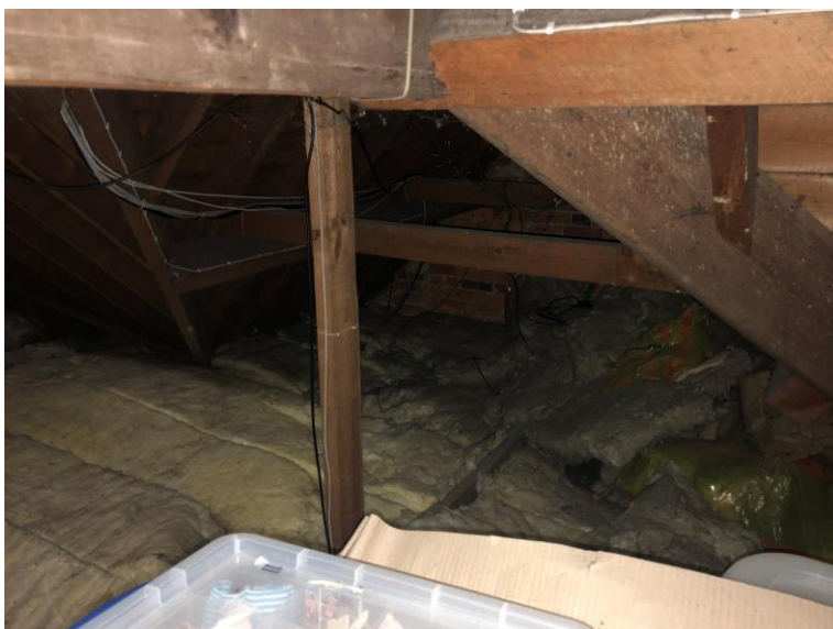
Plate 12. General view of the internal void space of the house.
