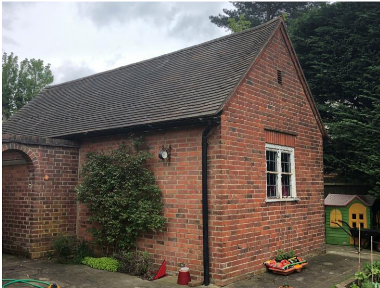
Plate 7. General view of the rear of the garage showing pitched roof.
