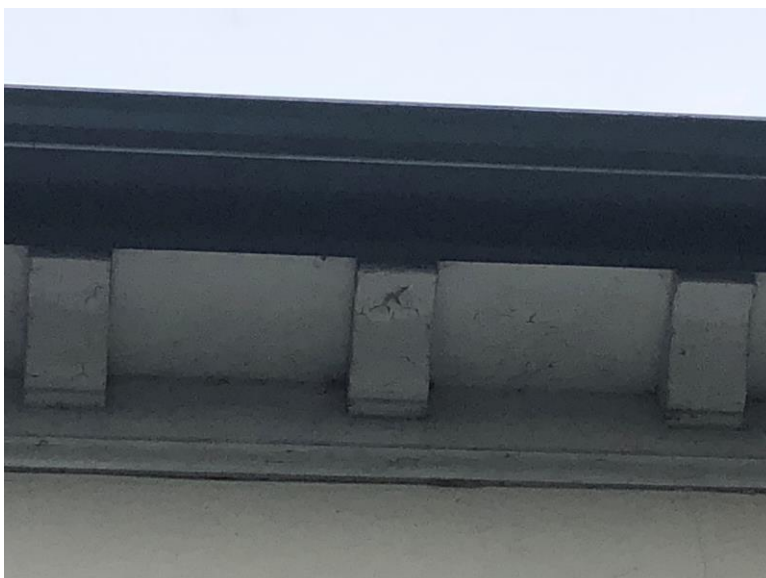
Plate 6. General view of the soffit and fascia.
