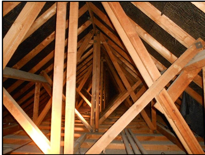
Photo 4.7: The internal roof space above the eastern half of the building.
