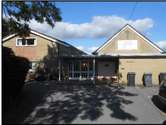
Photo 4.6: The Gate Church, south elevation.
