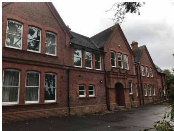
Photo 3- Central area of northern elevation
