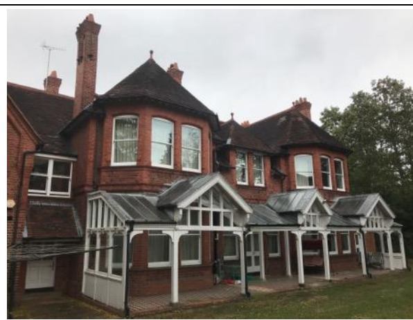
Photo 4 – Eastern end of southern elevation
