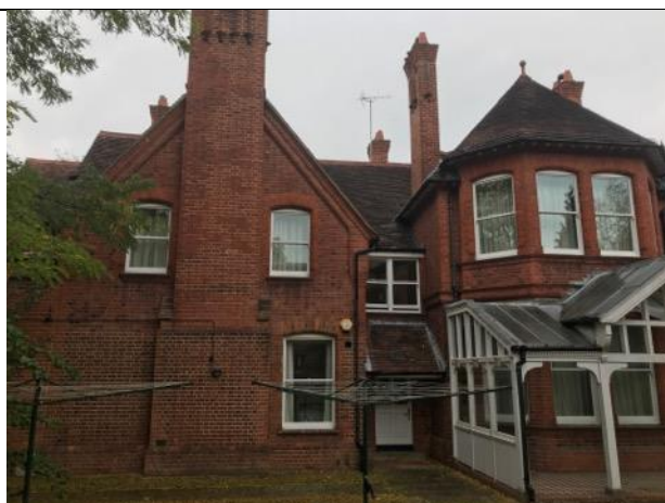
Photo 5: Western end of southern elevation
