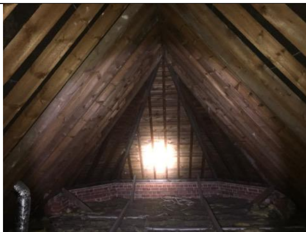
Photo 7: Inside sarked section of loft
