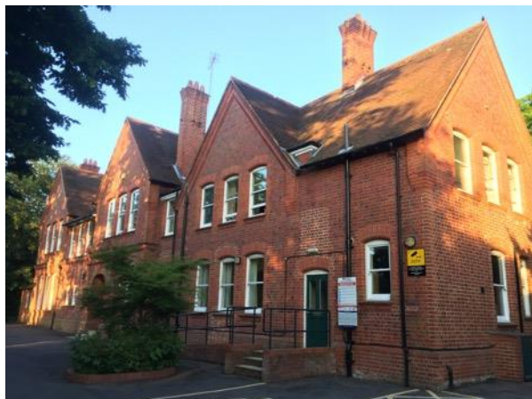
Photo 1 – Western end of northern elevation
