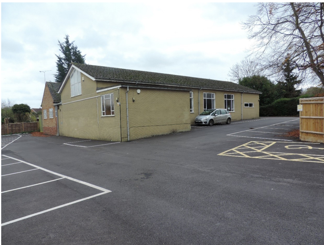
Existing poor quality church buildings from North West
