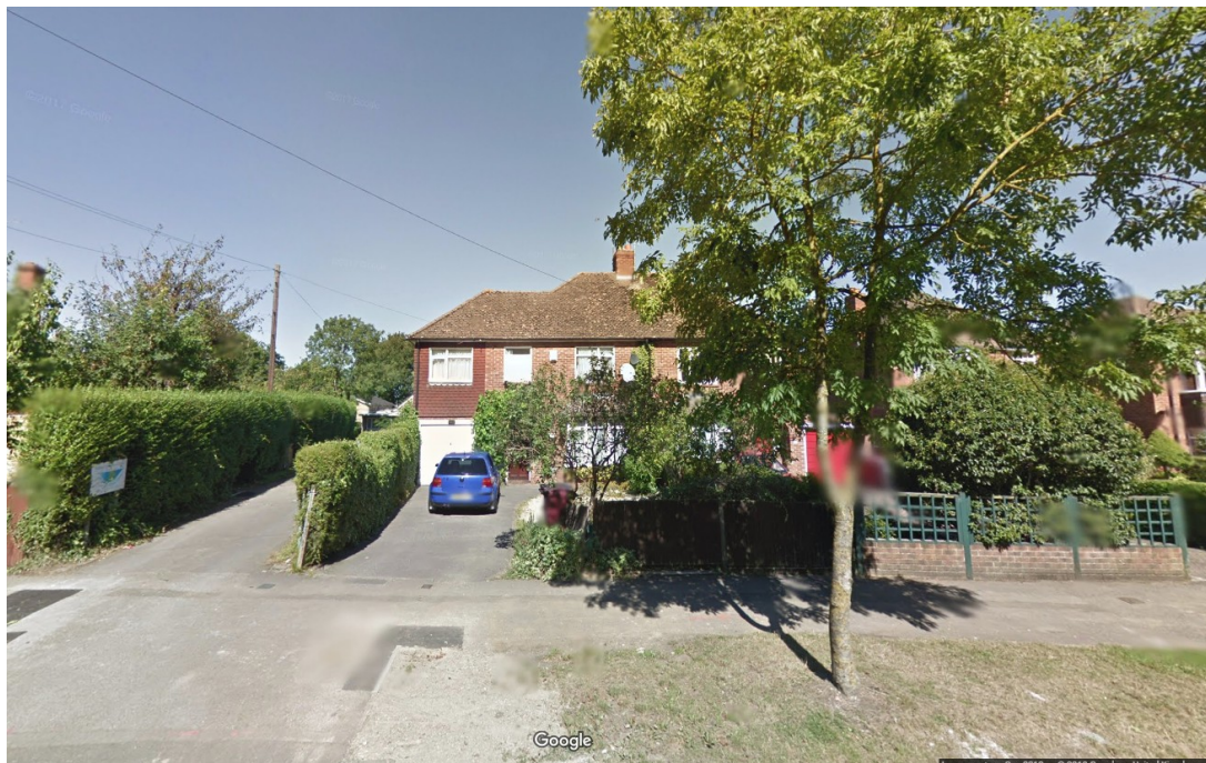
382 The Meadway – Two storey house with pitched roof. © 2018 Google
