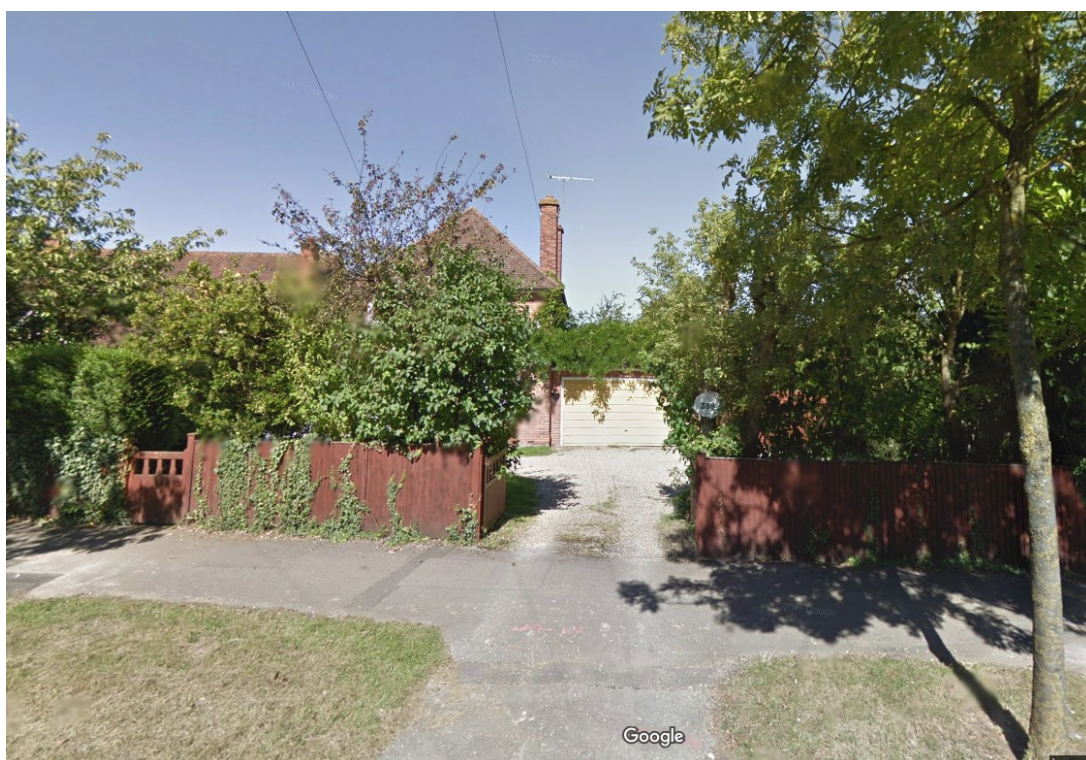
388 The Meadway – Two storey house with pitched roof. © 2018 Google
