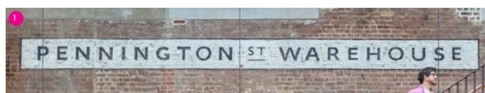
Precedent image - Painted sign-writing on brickwork facade
