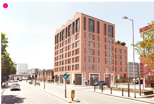
VIEW FROM NORTH OF CAVERSHAM ROAD
