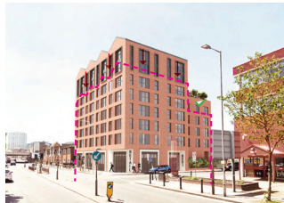
VIEW FROM CAVERSHAM ROAD
