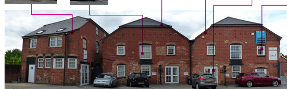
FORMER BREWERY BUILDING - INTERNAL FACADE
