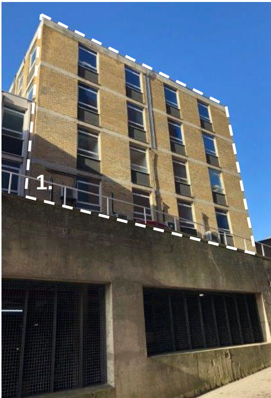
Rear Façade facing the Regus Building
