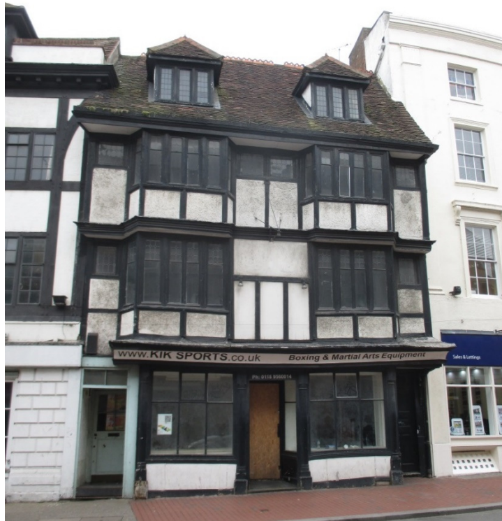
Figure 4.31: View of 27-28 Market Place
