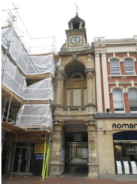
Figure 4.35: View of former Corn Exchange Arcade Entrance from the Market Place
