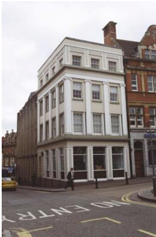
Figure 4.28: View of 52 Market Place and 10 High Street dated 2009 49
