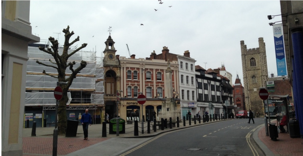
Figure 4.15: The historic buildings on the west side of the part-pedestrianised Market Place date from the 17 th -19 th centuries
