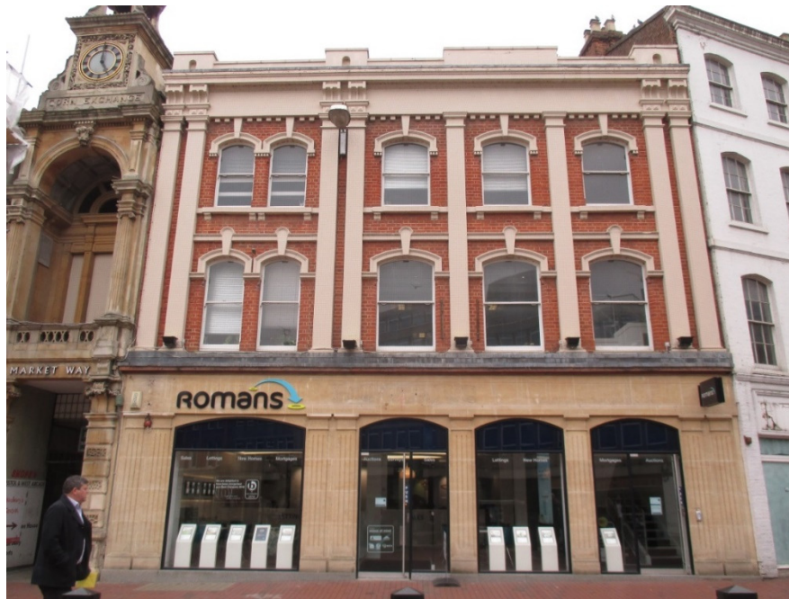
Figure 4.34: View of 33-34 Market Place
