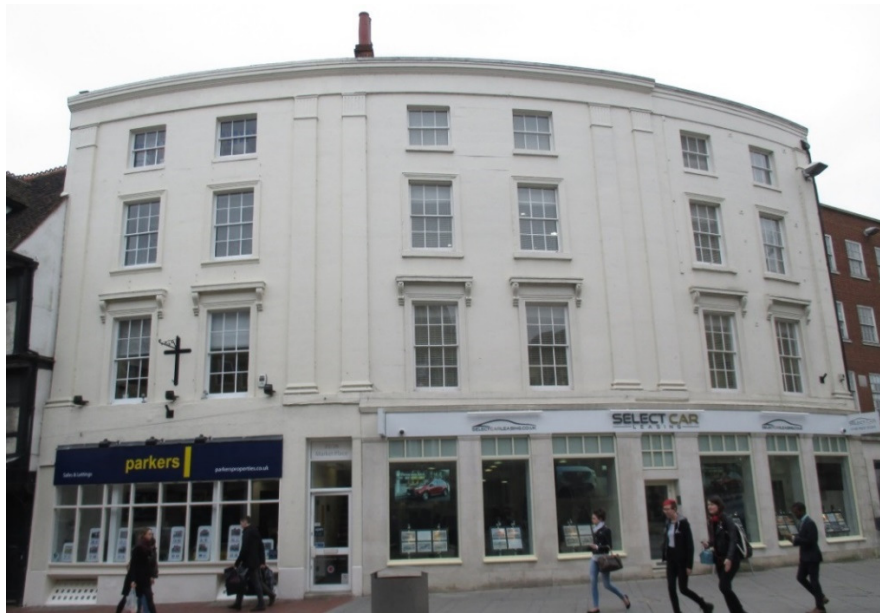
Figure 4.30: View of 23-26 Market Place
