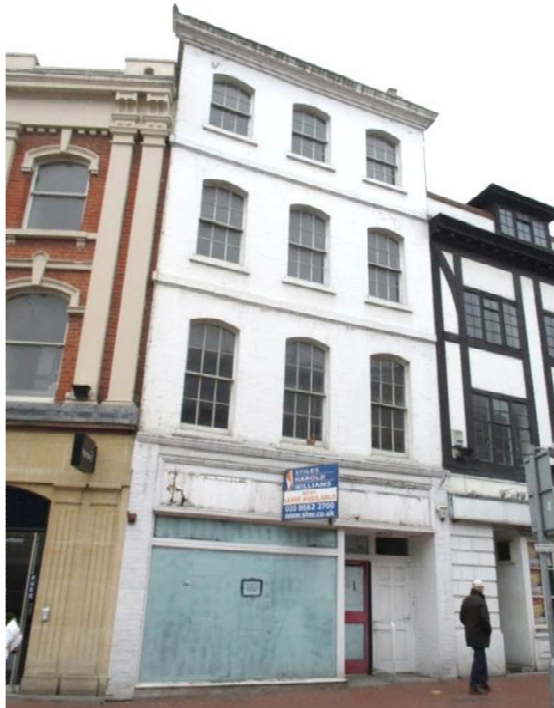
Figure 4.33: View of 32 Market Place
