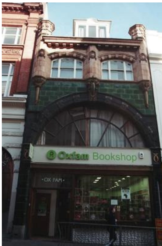
Figure 4.24: View of 8 High Street dated 2009 41
