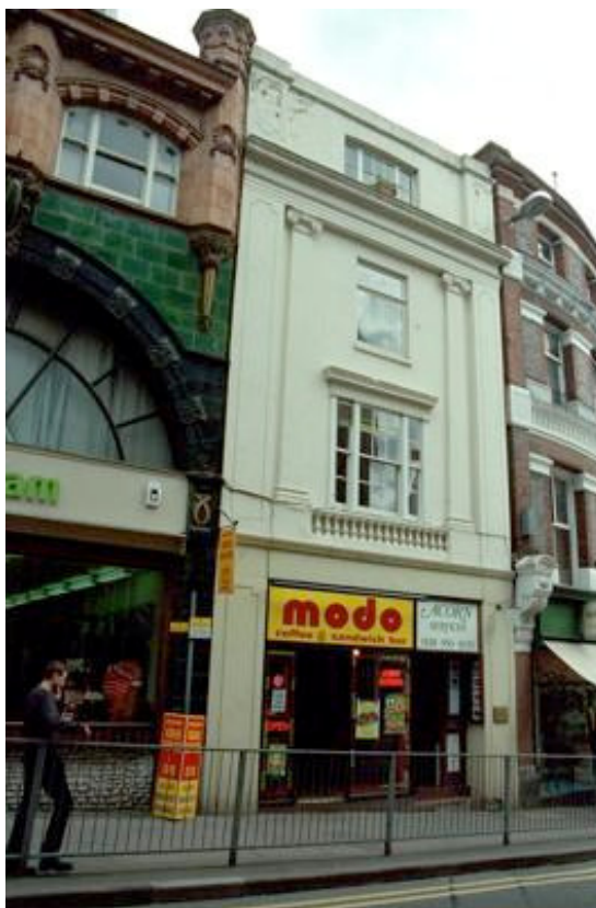
Figure 4.23: View of 7 High Street dated 2009 39
