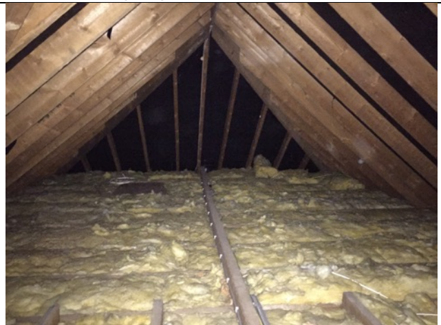
Photo 9 – Inside loft space looking south
