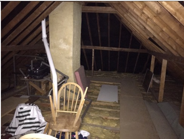
Photo 8 – Inside loft space looking west
