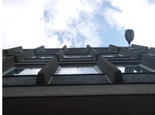
2. Front of the building viewed from the west.
