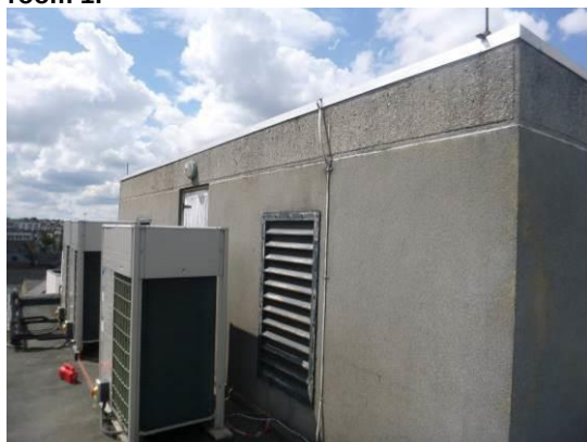
10. Tank room 2 with rendered walls with two large vents filled with wire mesh.
