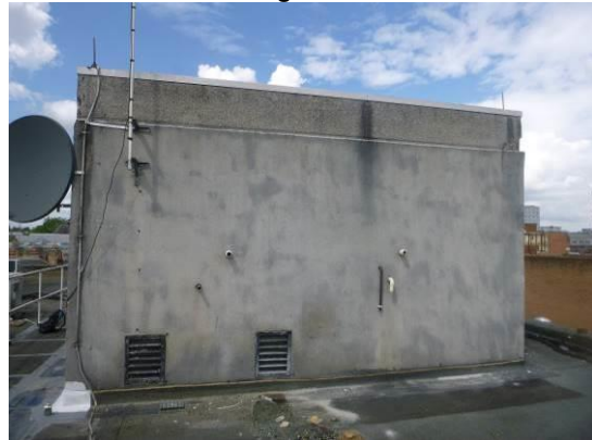
4. Tank room 1 with rendered walls and vents on the eastern side.
