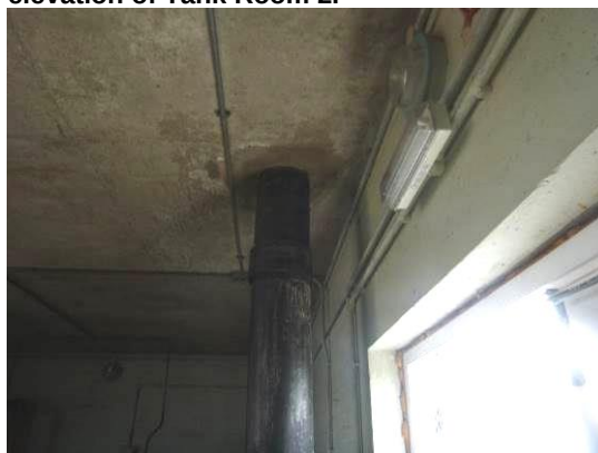
16. Roof lined with concrete in tank room 1.
