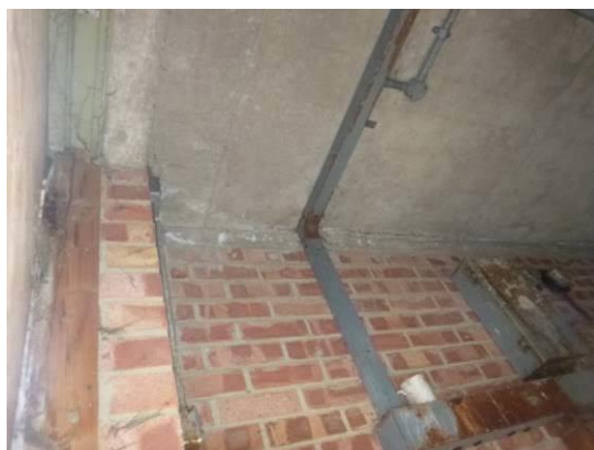
18. Roof lined with concrete in tank room 2.
