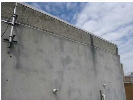
8. Fascia tight at the eastern elevation of tank room 1.
