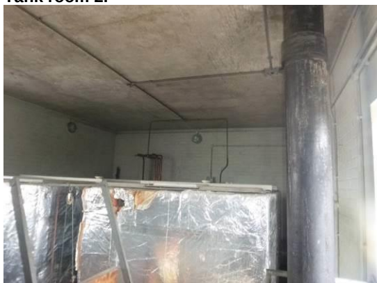
15. Internal view of tank room 1 with two water tanks.
