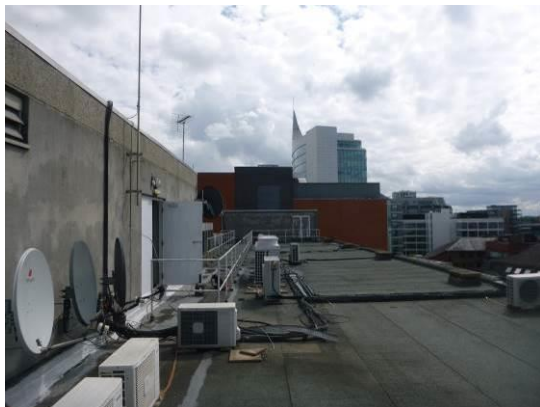
5. Vent and doorway on the southern side of Tank Room 1.
