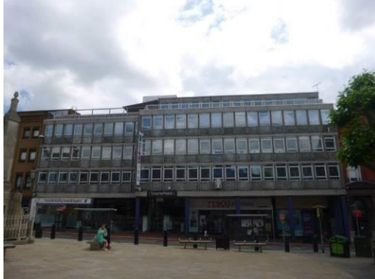
1. Front of the building viewed from the west.
