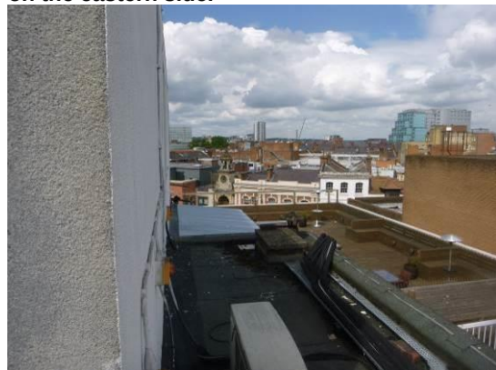
6. View of the northern side of the tank room which was not accessible.
