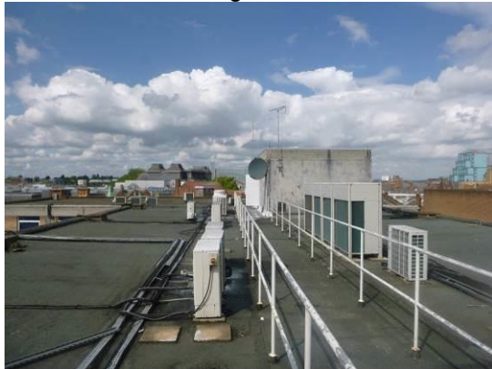
3. Bitumen felt tight on the floor of the roof.
