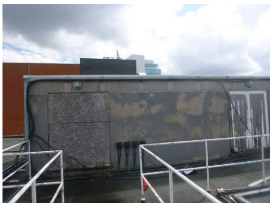
11. Boarded window on the western elevation of tank room 2.
