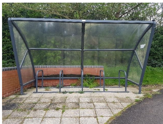
Current Cycle parking on site
