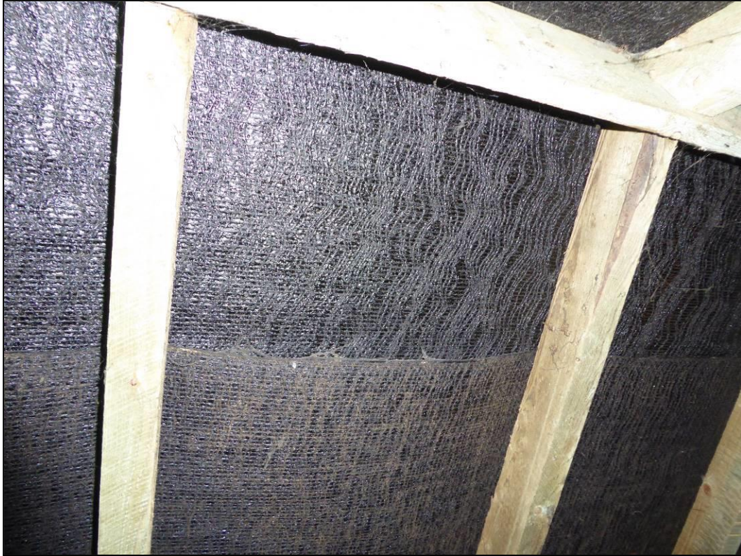
Figure 12. Example of bitumen lining. 9 Broomfield Road, Tilehurst. 24.09.19
