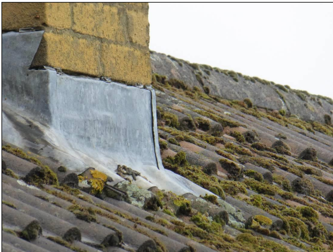
Figure 5. Example of lead flashing. 9 Broomfield Road, Tilehurst. 24.09.19
