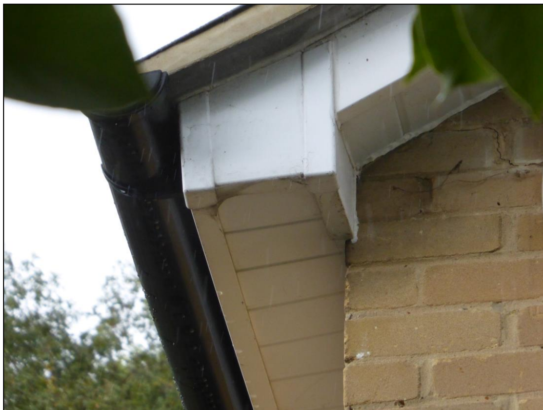
Figure 6. Soffits and fascias. 9 Broomfield Road, Tilehurst. 24.09.19
