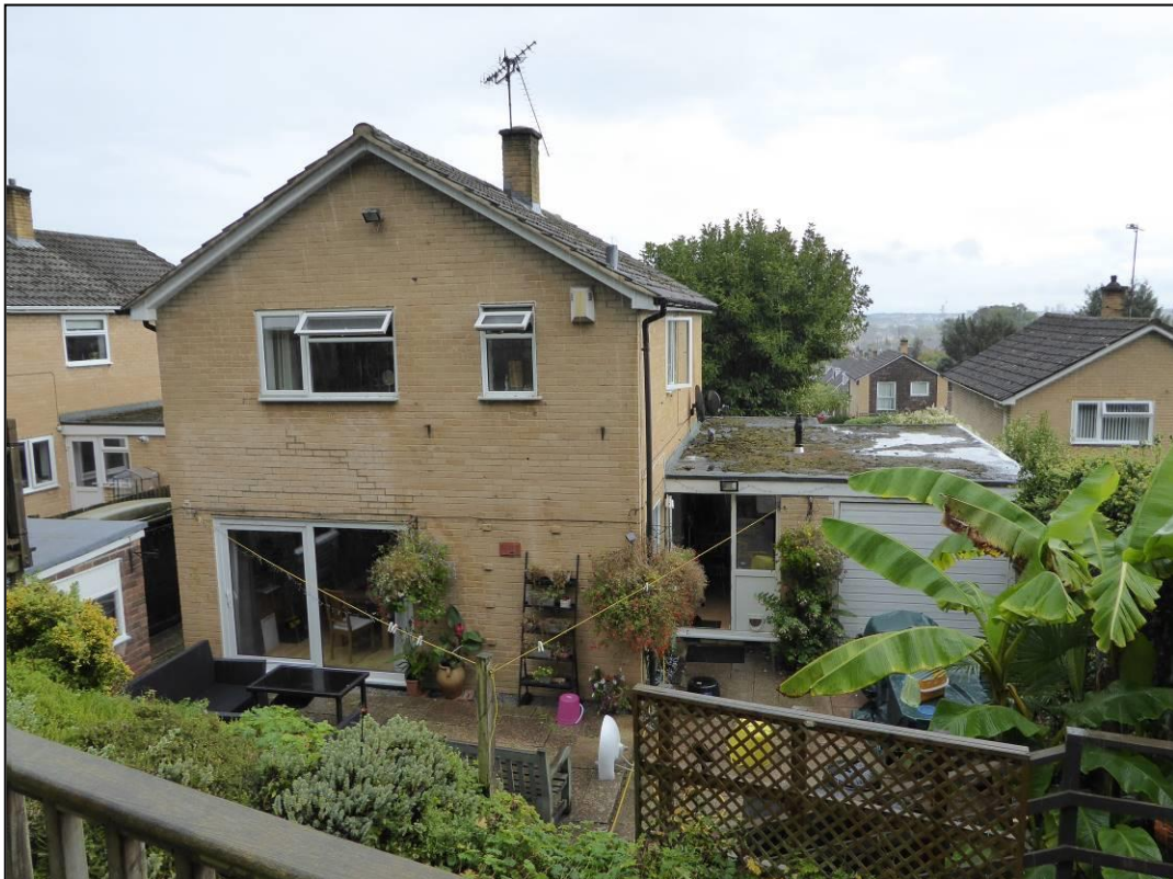
Figure 8. Rear view of the garage. 9 Broomfield Road, Tilehurst. 24.09.19
