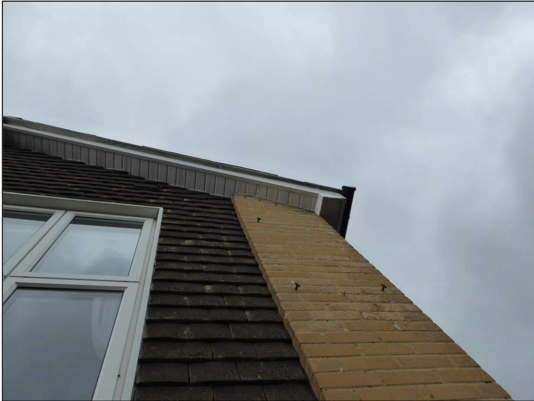
Figure 7. Hanging tiles. 9 Broomfield Road, Tilehurst. 24.09.19
