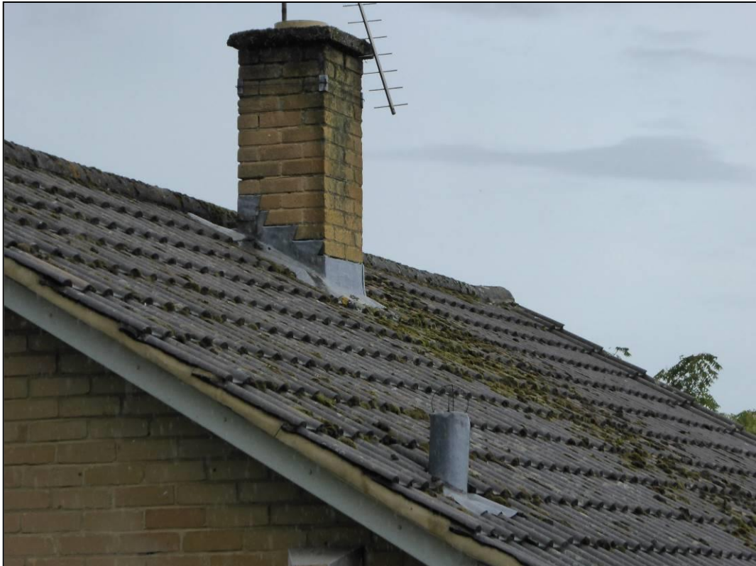
Figure 4. Example of roof tiles. 9 Broomfield Road, Tilehurst. 24.09.19
