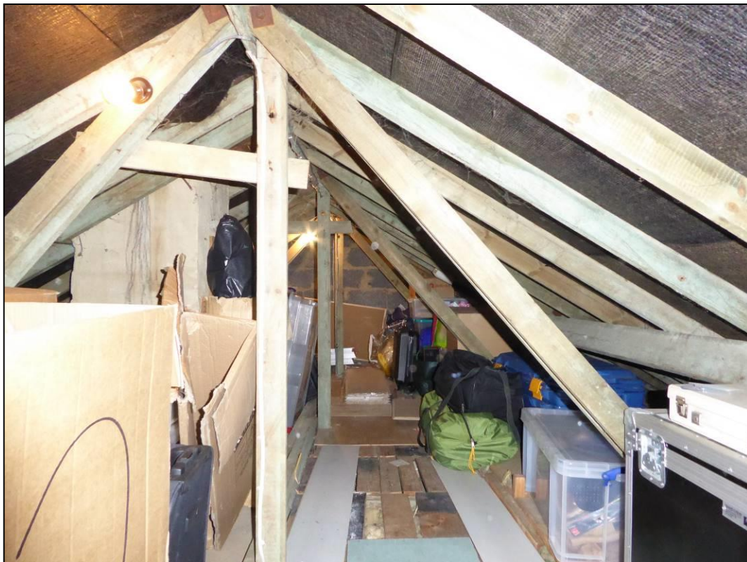
Figure 11. Example of loft space. 9 Broomfield Road, Tilehurst. 24.09.19
