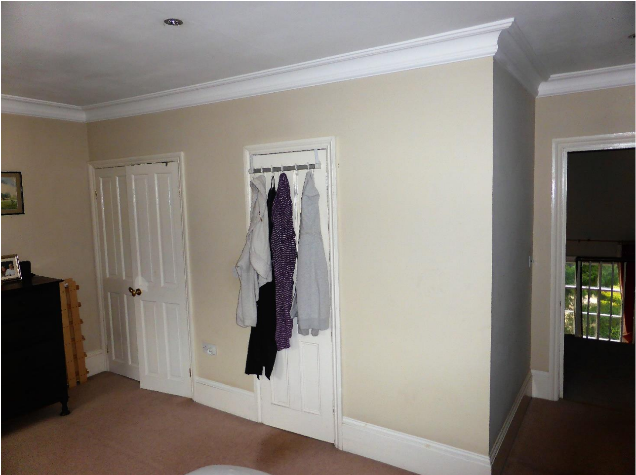
PHOTO 3. The door to the ensuite is centre frame, the relocated wardrobe is on the left and the relocated bedroom door on the right. The skirting from the removed first-floor partition wall appears to have been re-used to match existing. The cornice is most likely modern.
