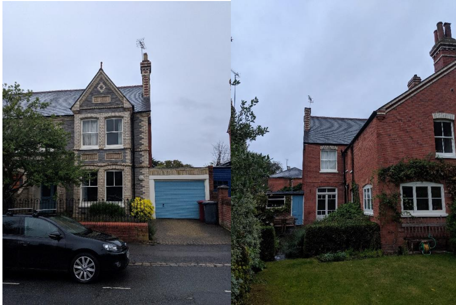
Figure 2. 55 Eastern Avenue. Front and Rear Elevations.
