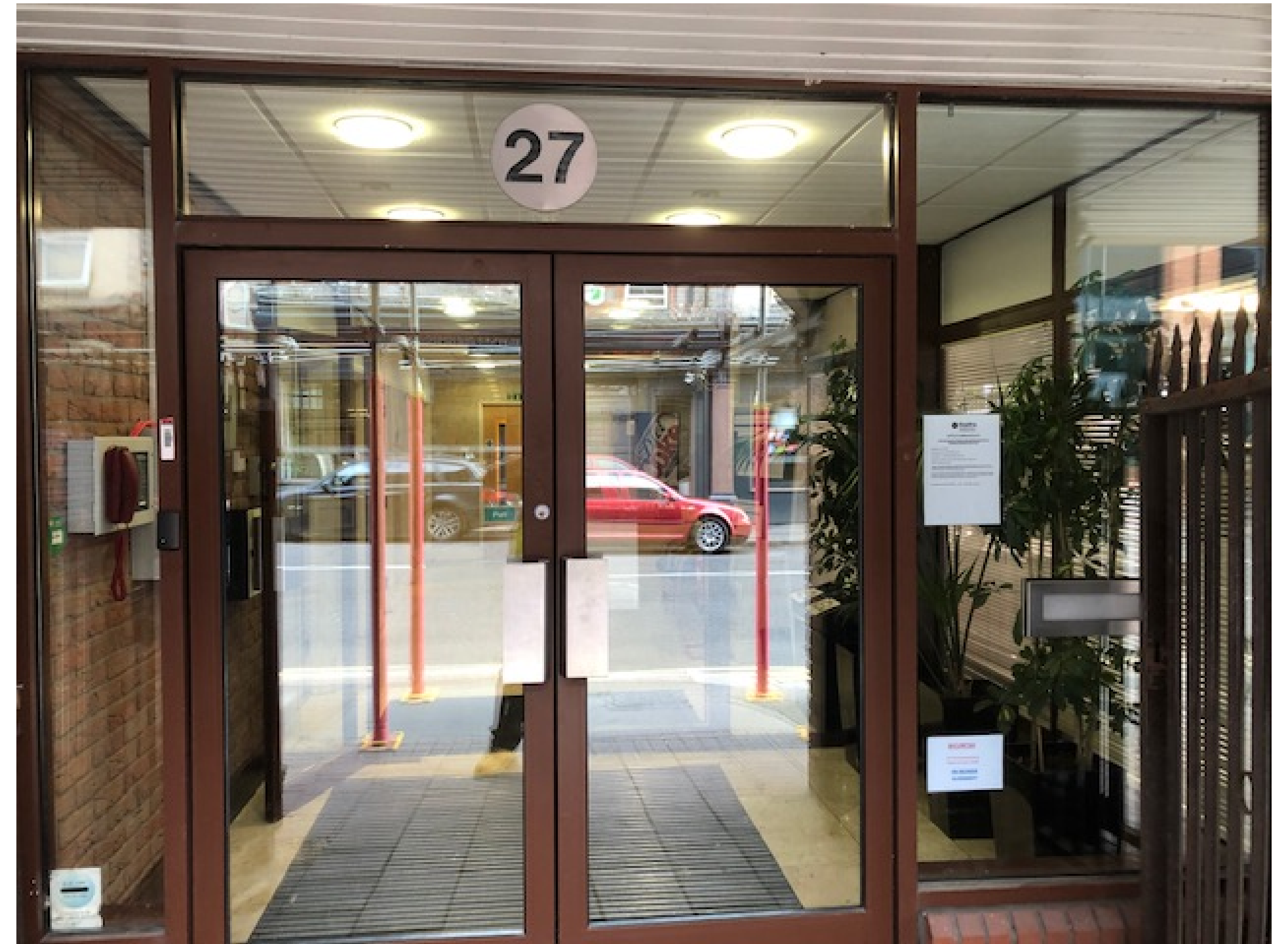
Picture no.1 Existing Main Entrance Doors
