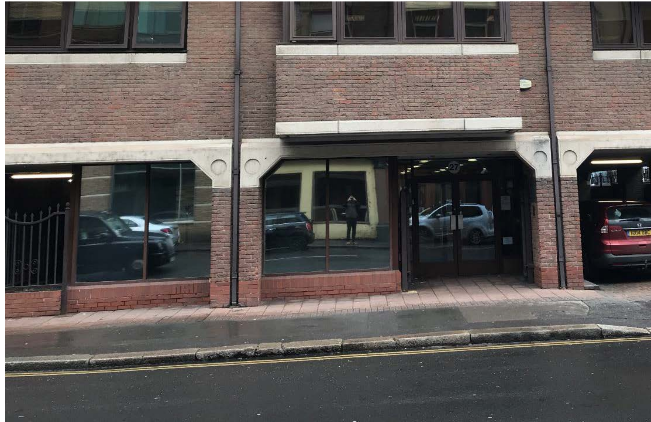
Existing Building Frontage
