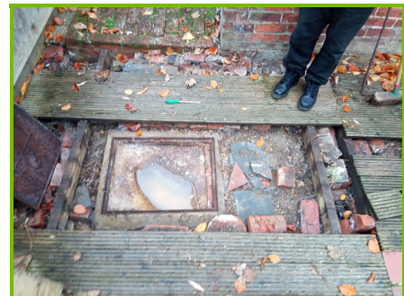
Fig 1.4: Manhole 1 (fully surcharged)
