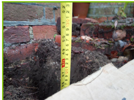
Fig 1.3: Depth of trial hole 1
