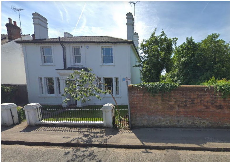
Above: Adjacent dwelling to plot 4 on Upper Redlands Road
