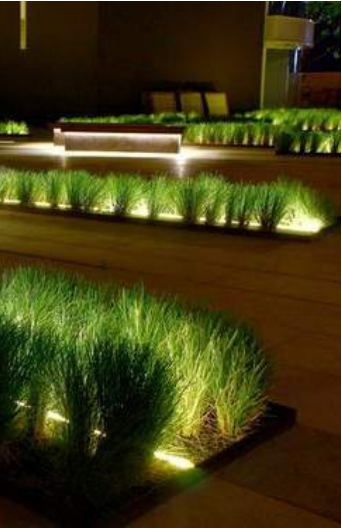
Tree and Shrub Lighting
