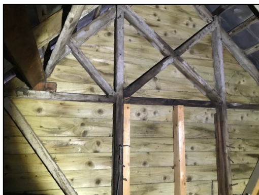
Figure 5 – internal view of weather boarding
