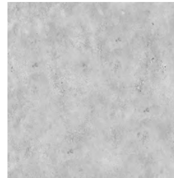
Exterior Fair-faced concrete column
