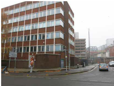
View of the Site from Greyfriars Road
