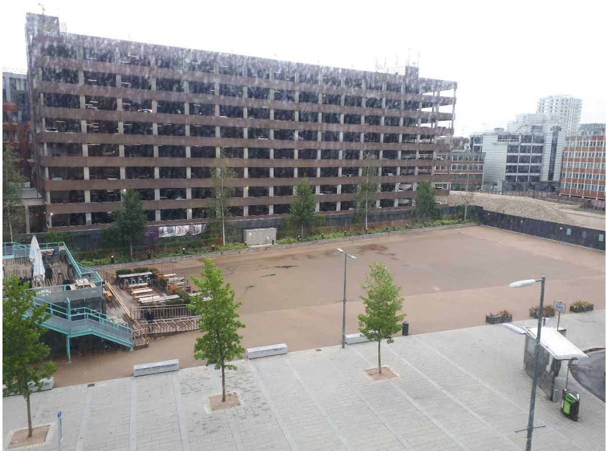
Photo 1: View from Reading Train Station looking south at NCP carpark and Temporary Events Space
