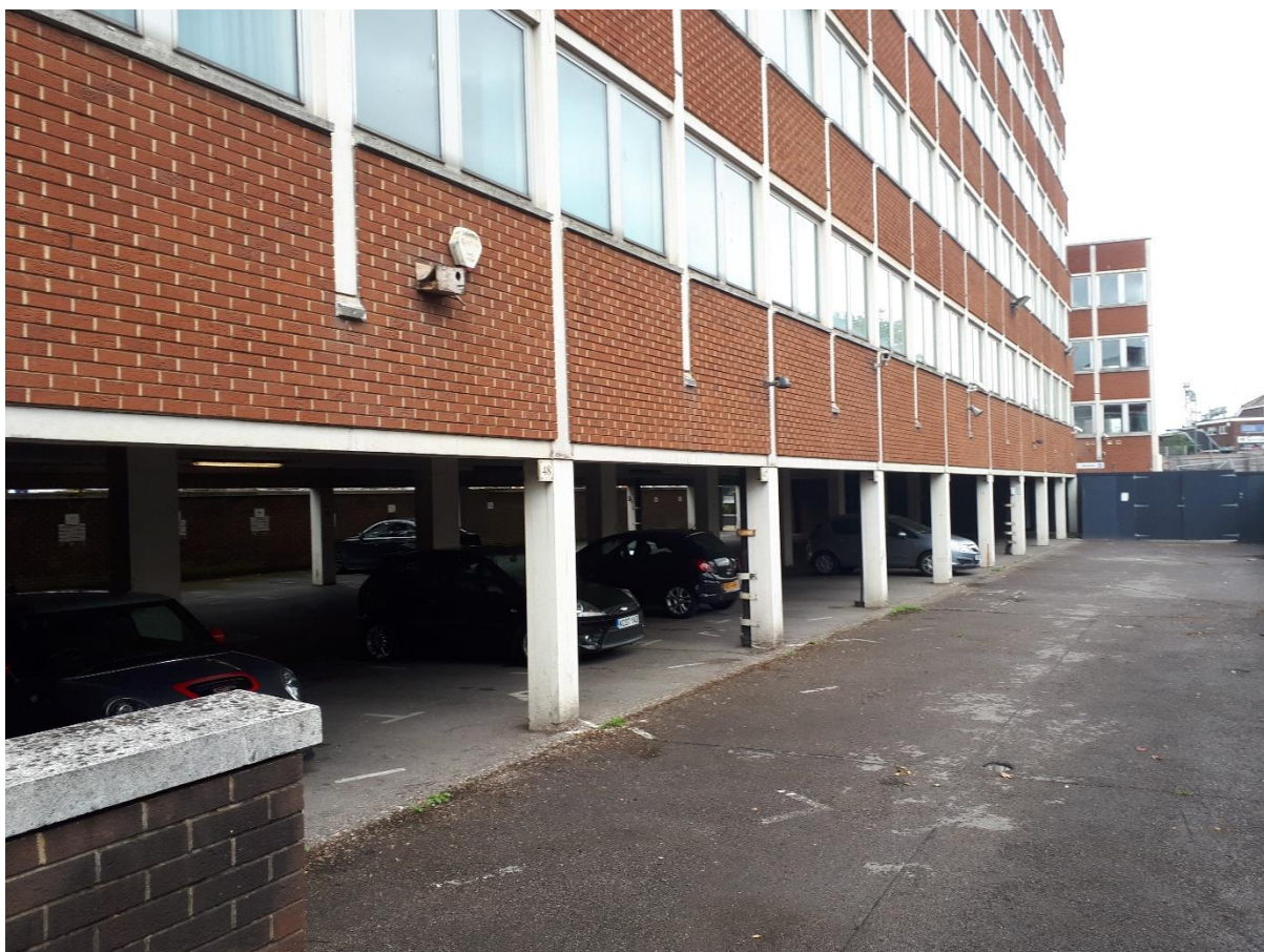
Photo 3: View Looking at carpark beneath Xaffinity House
