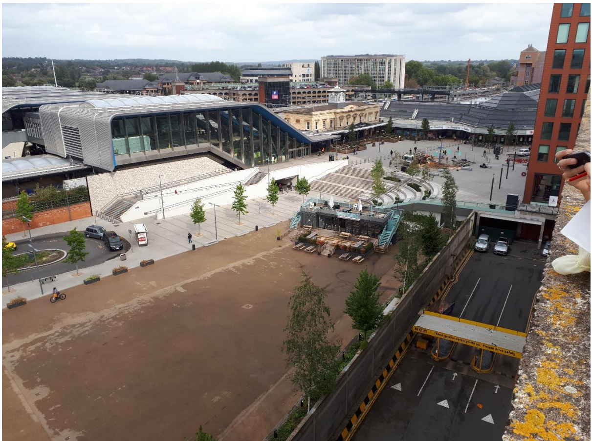
Photo 17: View looking north towards Reading Train Station, showing the Temporary Events Space.
