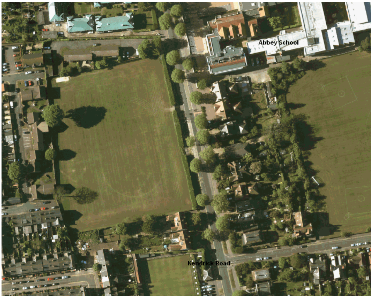
2010 Aerial Photograph PLANNING HISTORY
