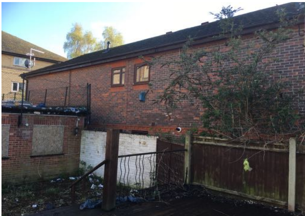
Photograph 6: Residential development located directly to the rear (south-west) of the Site
