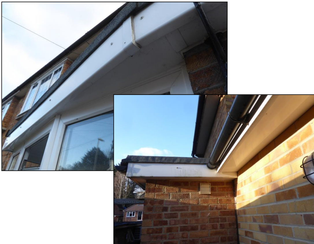
Figure 11. Sealed soffits and fascias on garage and side extension. 62 Rotherfield Way, Emmer Green. 10.01.20
