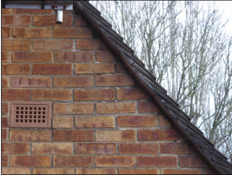
Figure 7. Example of sealed verges. 62 Rotherfield Way, Emmer Green. 10.01.20
