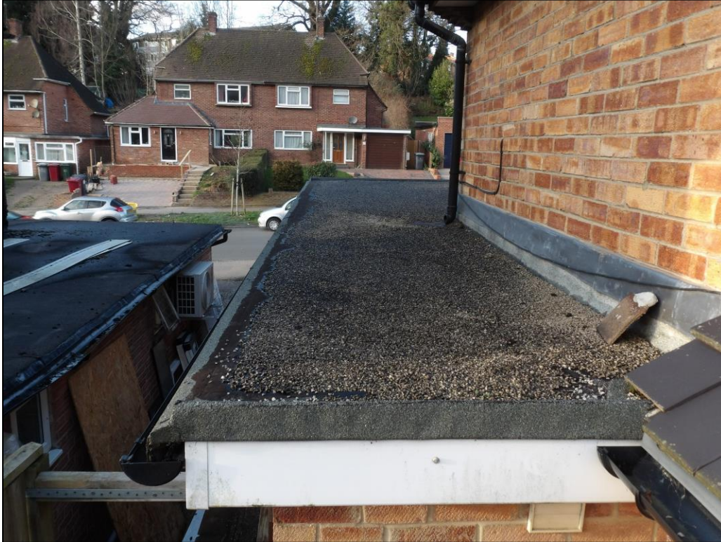
Figure 10. Flat roof over side extension and garage with sealed lead flashing. 62 Rotherfield Way, Emmer Green. 10.01.20
