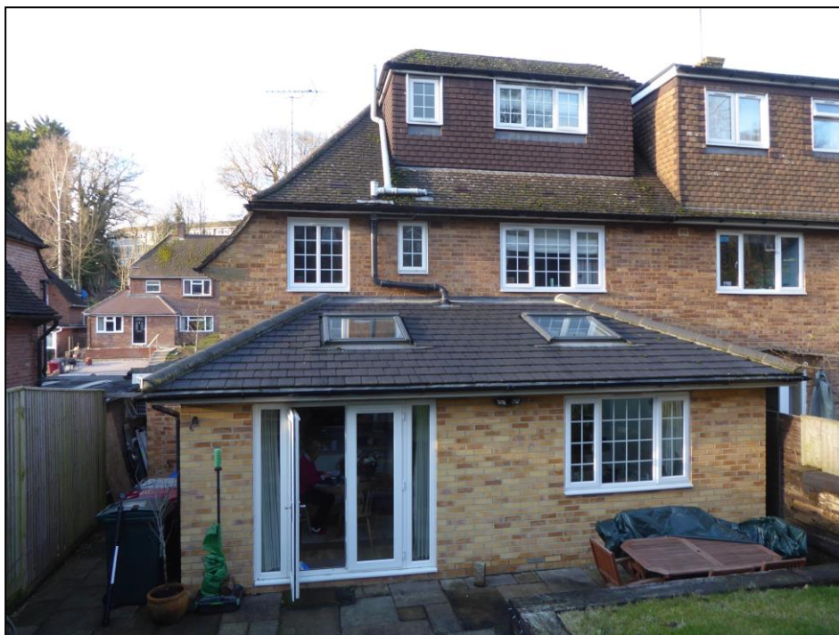
Figure 4. Example of roof structure. 62 Rotherfield Way, Emmer Green. 10.01.20
