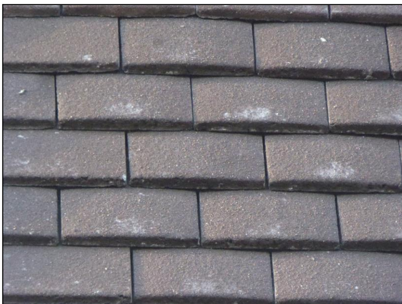
Figure 9. Tight fitting hanging tiles. 62 Rotherfield Way, Emmer Green. 10.01.20
