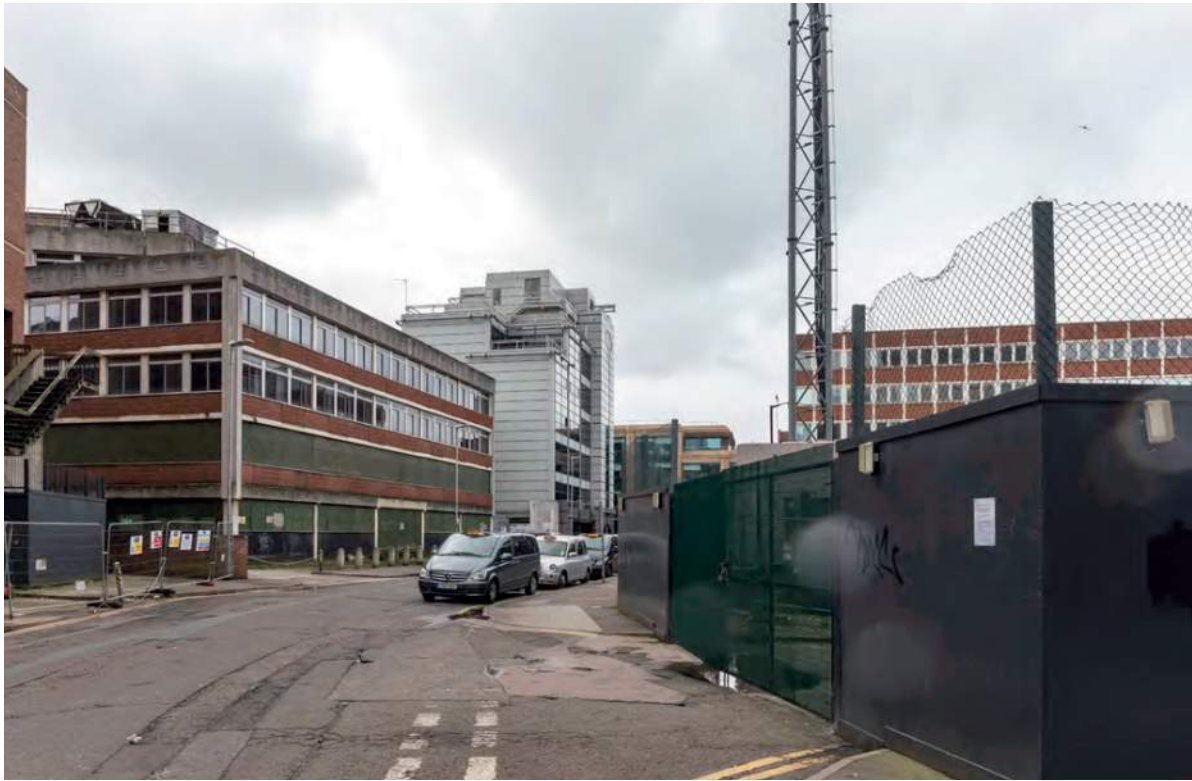
View from Garrard Street looking west towards the site.
