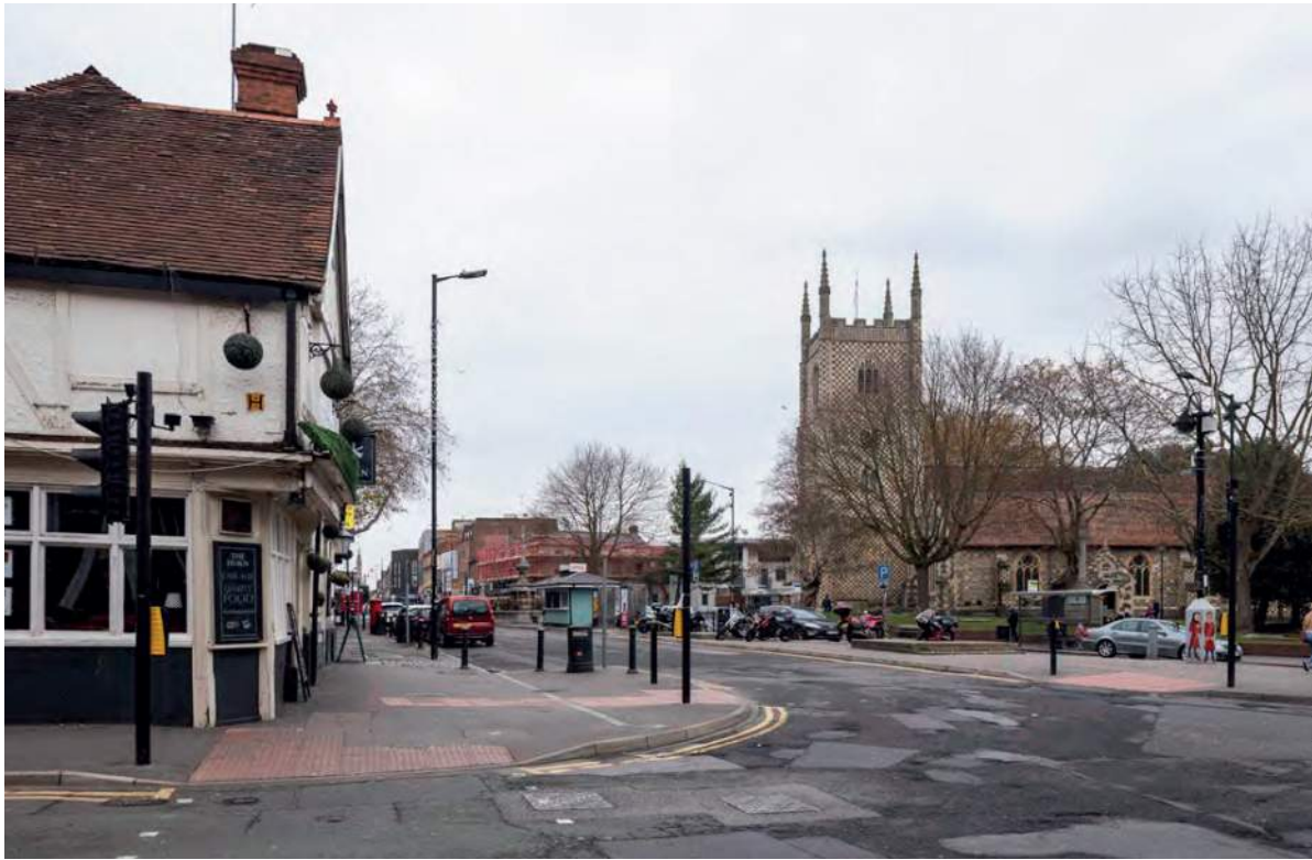
View from the junction of Castle Street and St Mary's Butts looking north-east towards the site.
