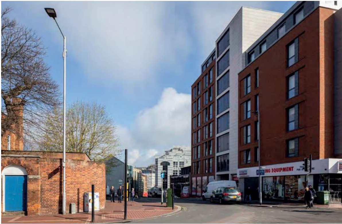
View from Junction of Friar Street and Greyfriars Road looking northeast towards the site.
