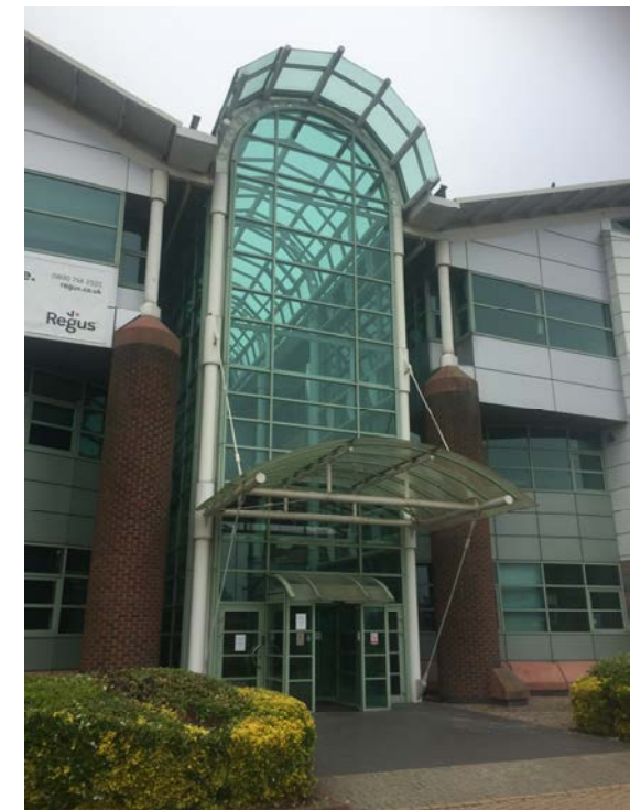
Main entrance screen
