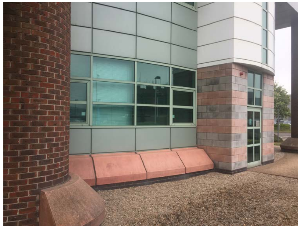
Ground floor windows and escape doors
