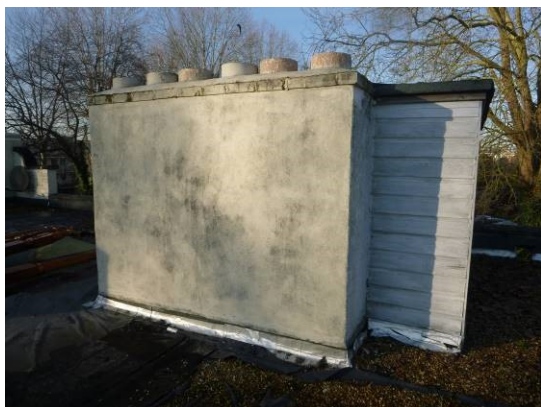
7. Flashing tape along base of chimney and store room (viewed from roof).
