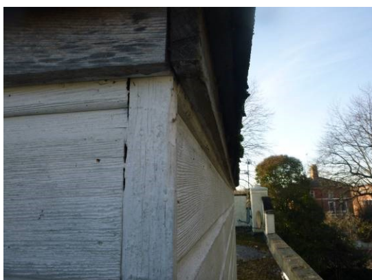
11. Tight timber barge boards and painted cladding on store room (viewed from roof).
