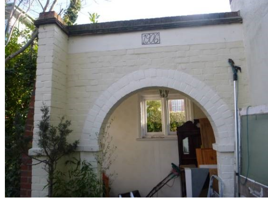
14. Loggia section at rear of side extension (north elevation).
