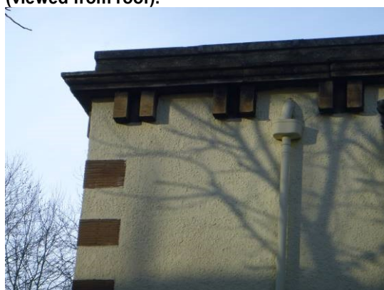
12. Intact stonework beneath roof parapets (rear elevation).
