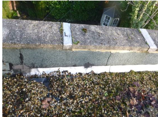
6. Flashing tape along roof parapets (viewed from roof).
