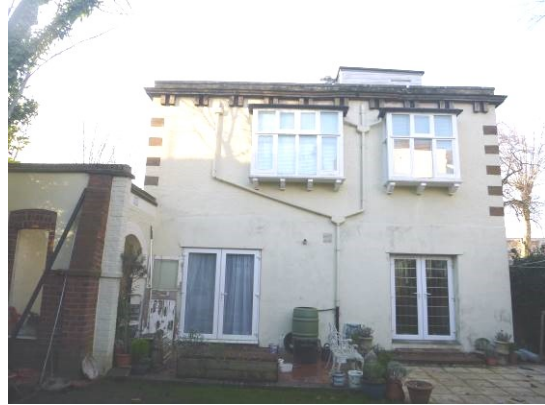
2. Rear of property viewed from east.
