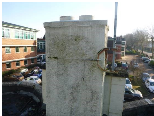
8. Southern chimney (viewed from roof).
