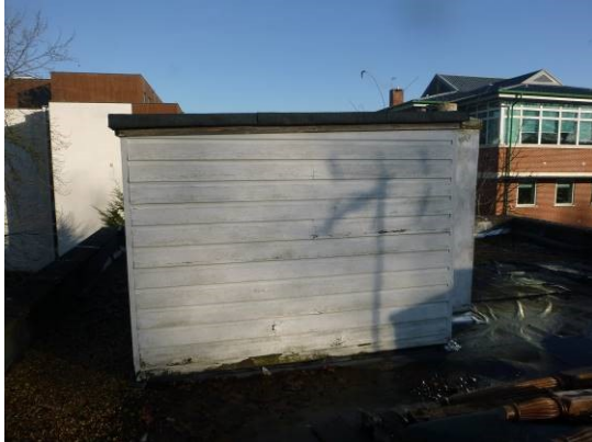
3. Store room on top of roof (viewed from roof).
