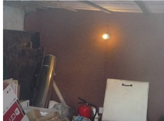
16. Boarded walls in store room.
