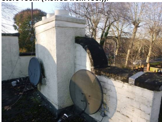
9. Northern chimney (viewed from roof).
