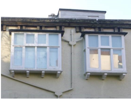
13. Intact oriel windows (rear elevation).
