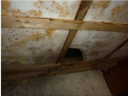
15. Roof of store room insulated with polystyrene.
