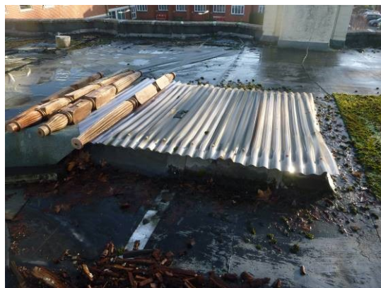
10. Rooflight covered with corrugated uPVC (viewed from roof).
