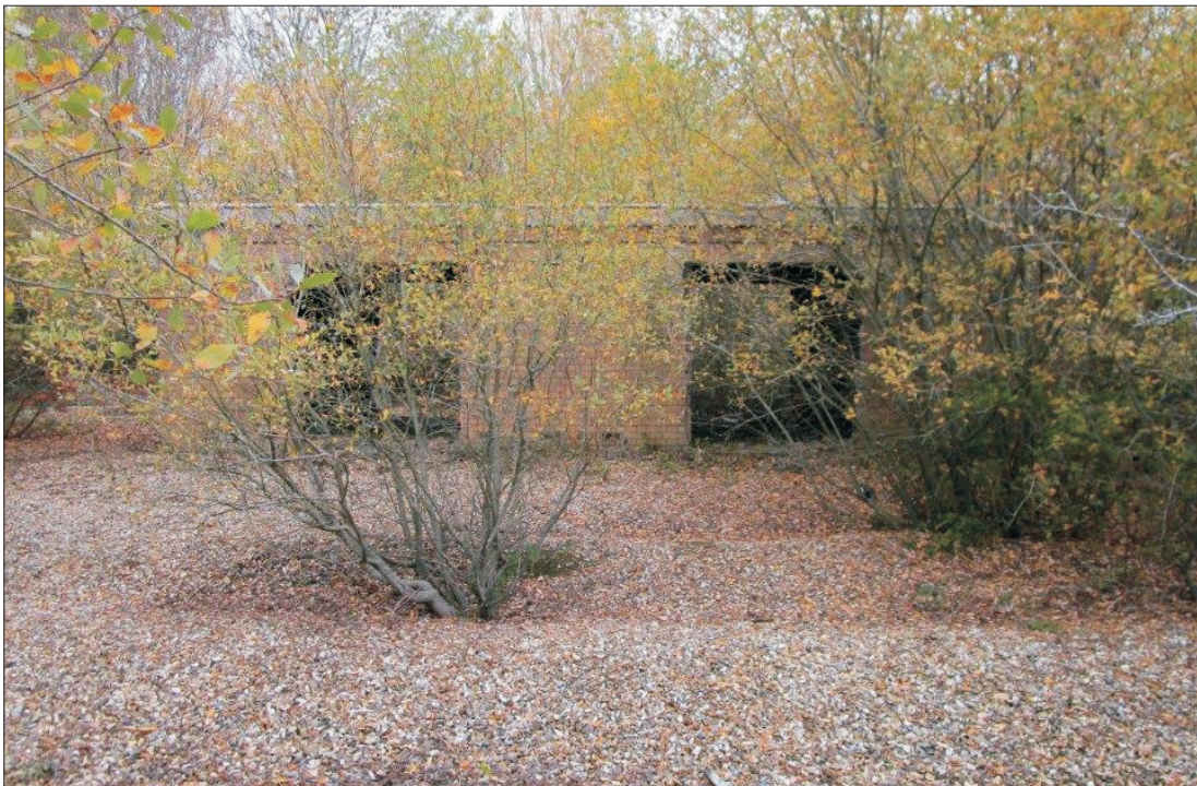
PHOTOGRAPH 4: Building B1 and Surrounding Gravel
