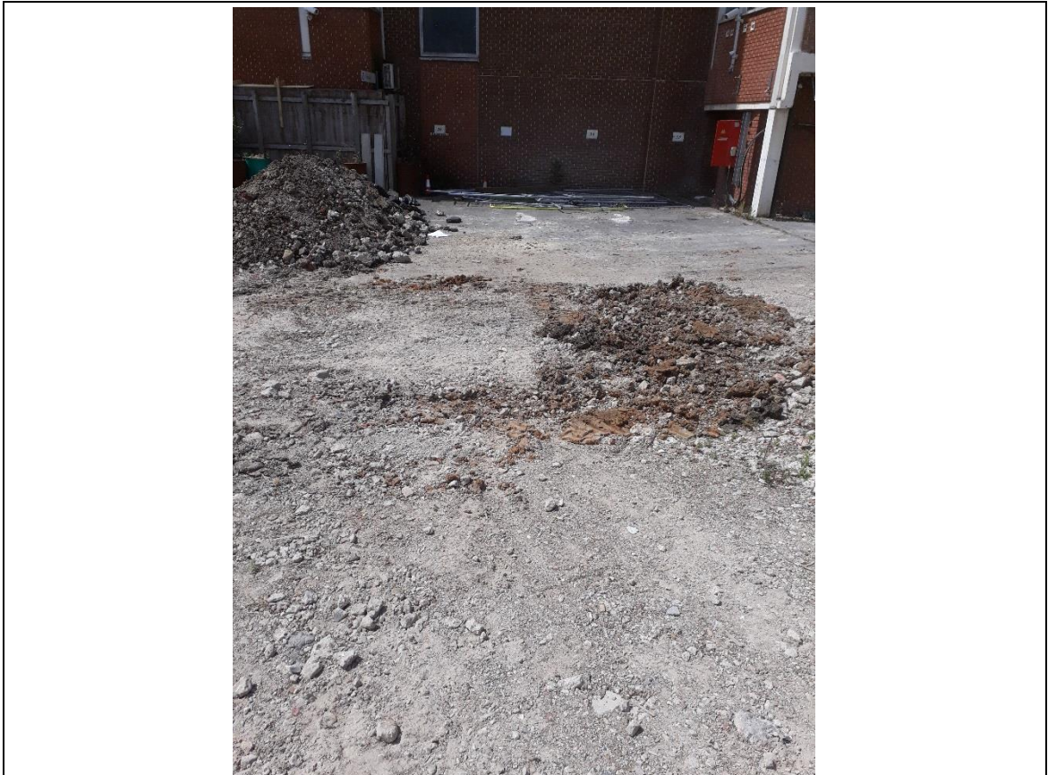
Trial Pit: TP205 Backfill
