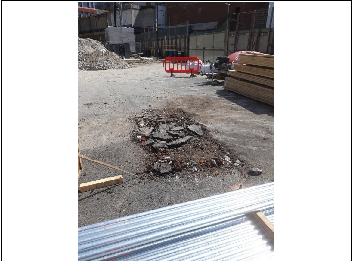
Trial Pit: TP206 Backfill
