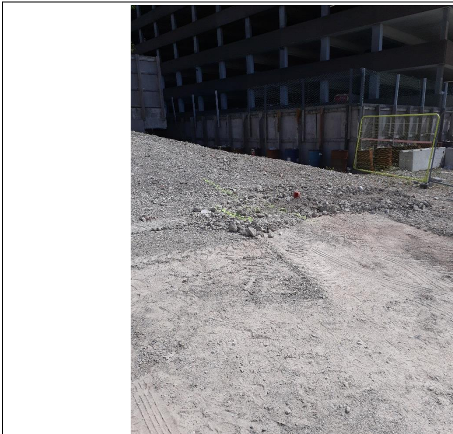
Trial Pit: TP209 Backfill
