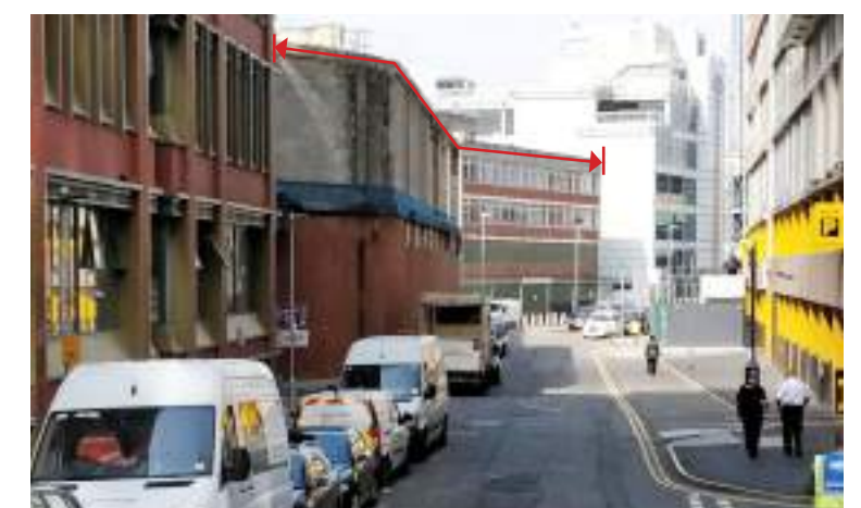
Existing buildings facing Garrard Street, viewed from the east
