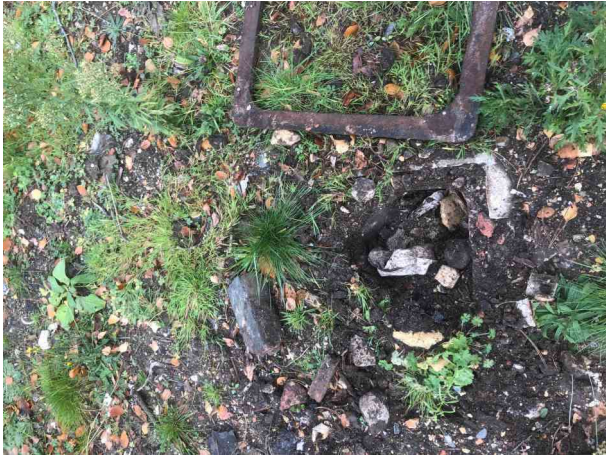
Overview 2X_eefc8aa2-ef4a-4f57-b26c-8d9556696361_20191125_1903 43.jpeg, 0.00 m General remark, Manhole backfilled
