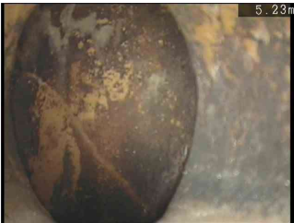
F1X_5b72d655-f6e5-40ba-907f-d260f462b7c9_20191125_180005_275.jpg, 00:01:19, 5.23 m Fracture, longitudinal at 10 o'clock, Junction fractured
