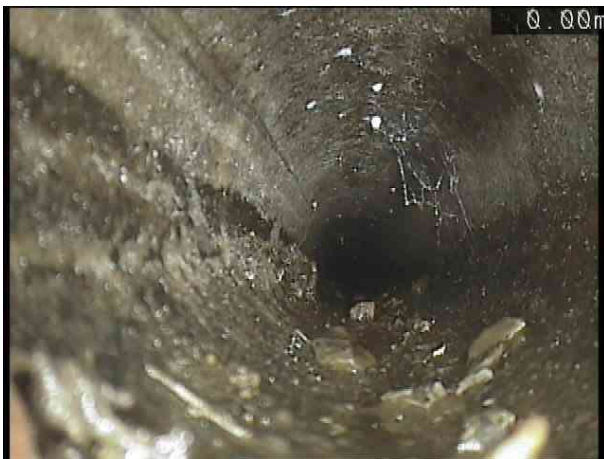
Main LineX_4626f6d1-c223-48ac-9156-7b01283da7fd_20191125_145059_254.jpg, 00:00:02, 0.00 m Water level, 0% of the vertical dimension
