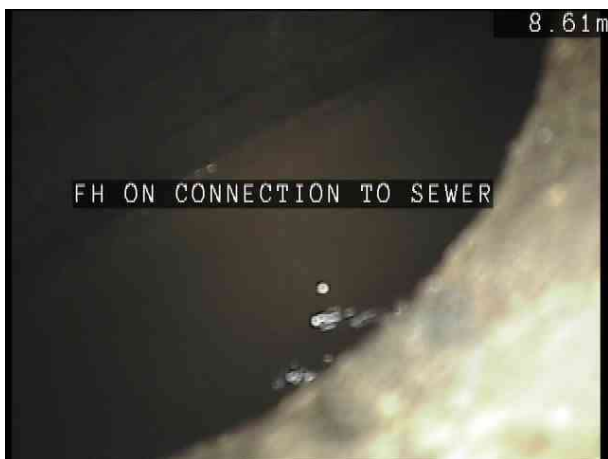
F1X_367a38c3-5331-4139-8343-bfec51ef7a60_20191125_180257_132.jpg, 00:02:08, 8.61 m Finish node type, major connection without manhole, reference number: Sewer, FH on Connection to Sewer
