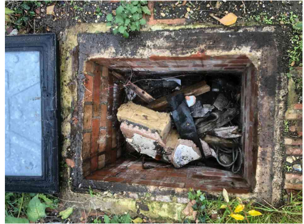
Overview 3X_f34978a8-fce4-4c84-b07a-6b0ad8b078fd_20191125_1907 17.jpeg, 0.00 m General remark, Manhole backfilled
