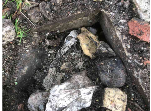
Overview 2X_5649e633-bffe-4f89-ac61-9344dc957eeb_20191125_1904 43.jpeg, 0.00 m General remark, Manhole backfilled
