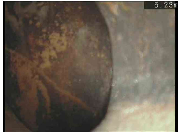
F1X_36b79757-2361-402a-a0cf-dfdcf61e96b8_20191125_175725_826.jpg, 00:01:19, 5.23 m Line deviates down
