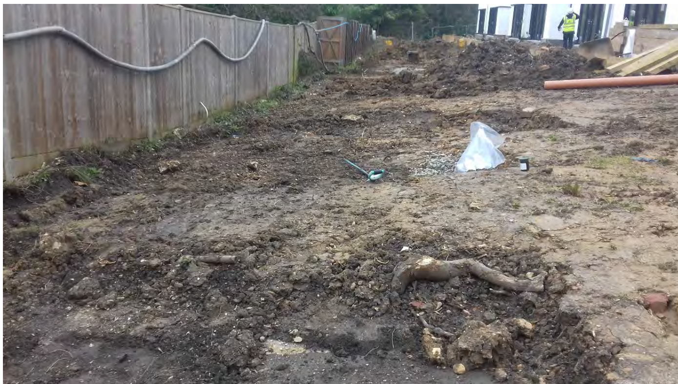
Above, the plot 1-4 garden area excavated to about 0.6m below finished ground level
