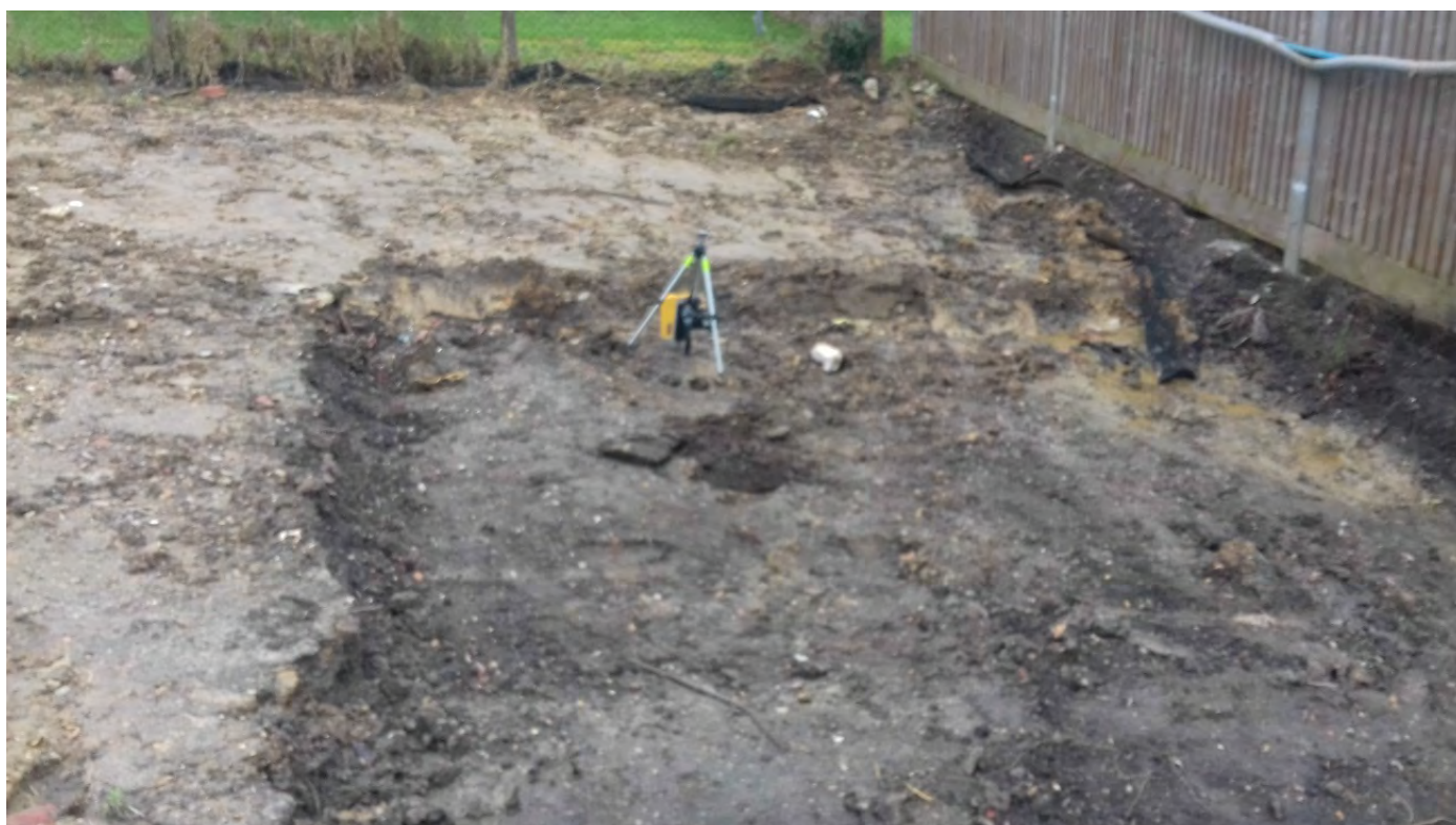
Above, XRF analyser set up and testing the dark brown ashy topsoil layer.
