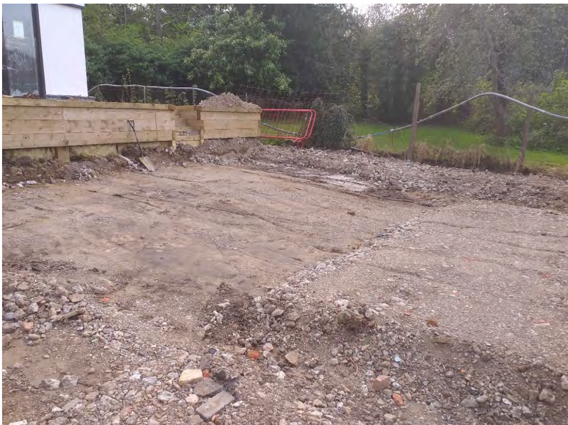
Above and below, the plots 1-4 garden area after additional excavation and placement of part of the break layer specified in the report.
