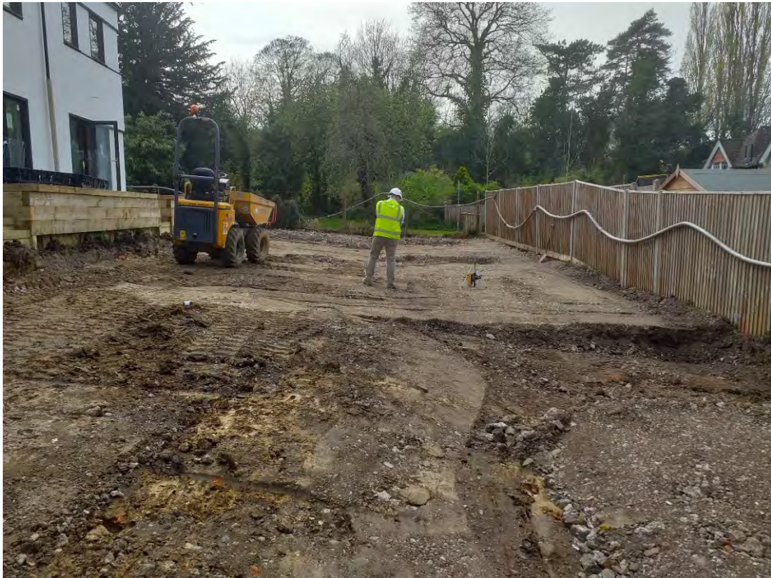
Above and below, the plots 1-4 garden area after additional excavation and placement of part of the break layer specified in the report.
