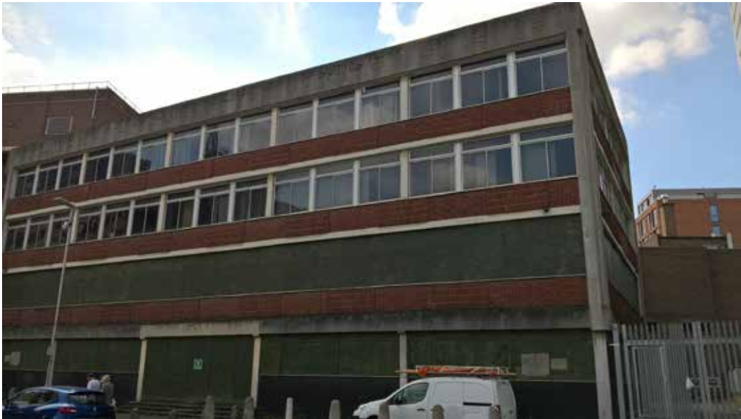
View of Buildings looking south from Garrard Street
