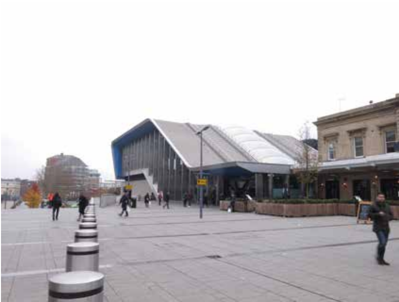
Reading Station to the north of the Site
