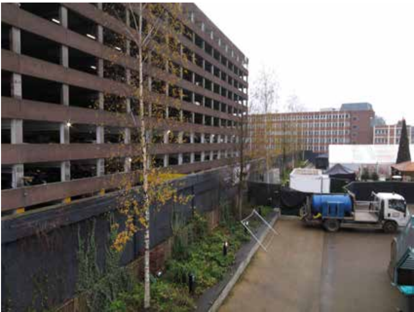
View of NCP Car Park
